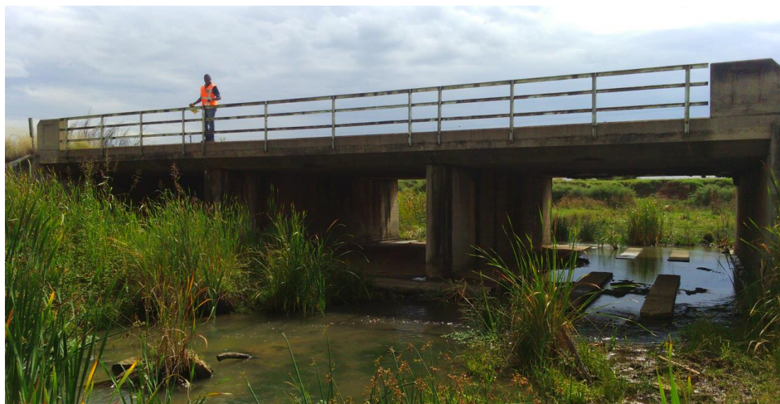
Figure 8-2: Bridge Upstream of RTSF (Bridge 2)
