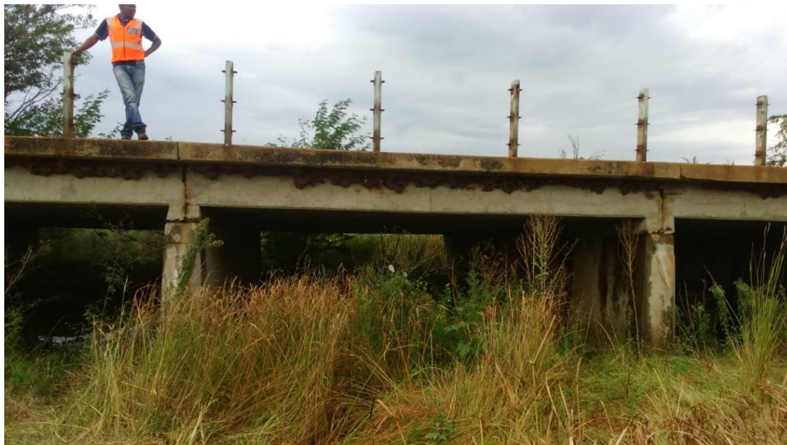
Figure 8-1: Bridge Downstream of RTSF (Bridge 1)
