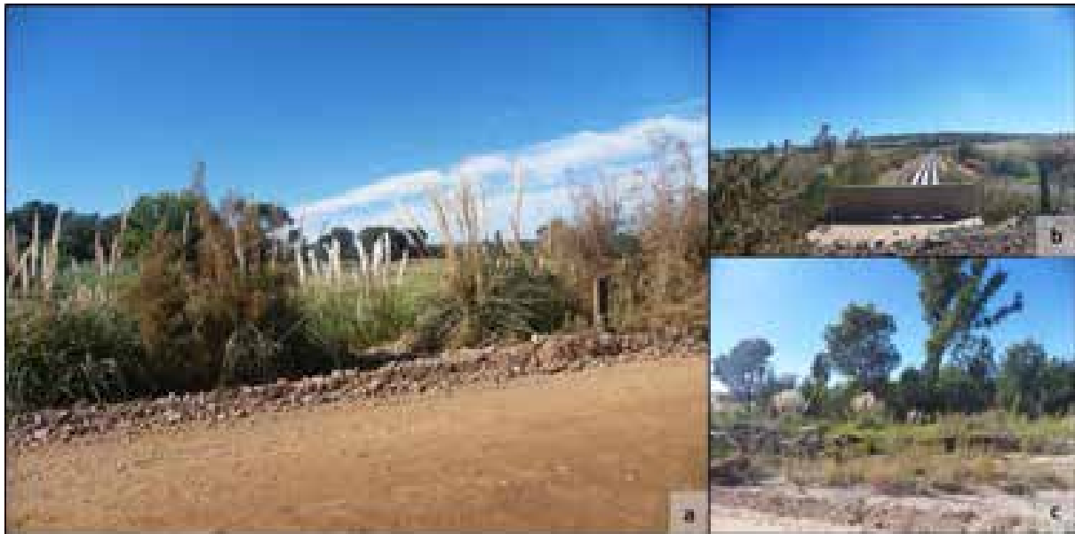
Figure 7-18: Wetland 14b (CVB) photos: a) stretch of wetland impacted by road crossings and the exotic species Pampus Grass ( Cortaderia selloana ); b) impacts of pipeline servitudes through the wetland; and c) general condition of the wetland with multiple impacts
