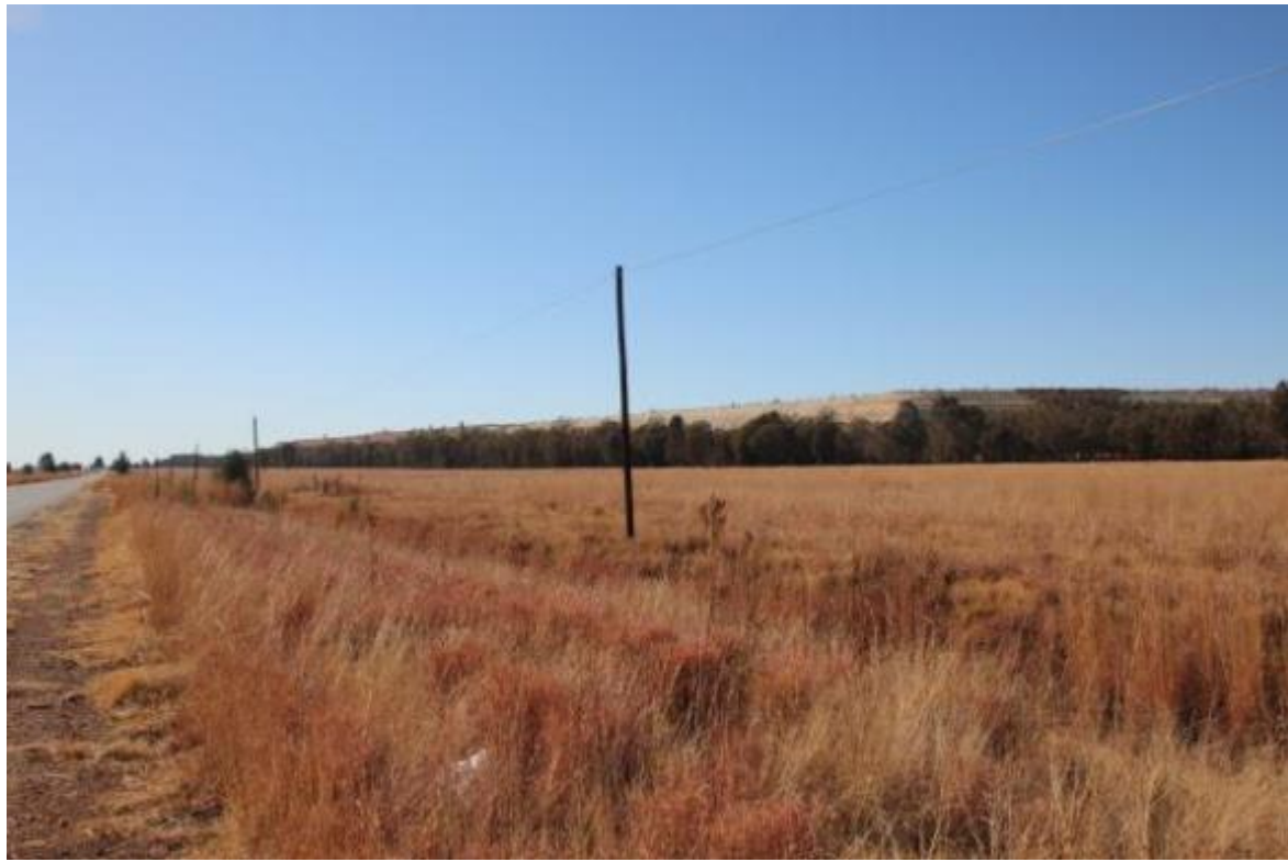
Figure 8: View of Driefontein 3 TSF from the R501 Regional Road
