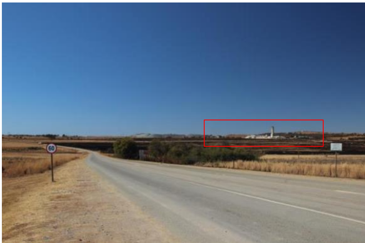
Figure 4: View of Plant and Shaft Infrastructure in the Kloof MRA from 2.4 km
