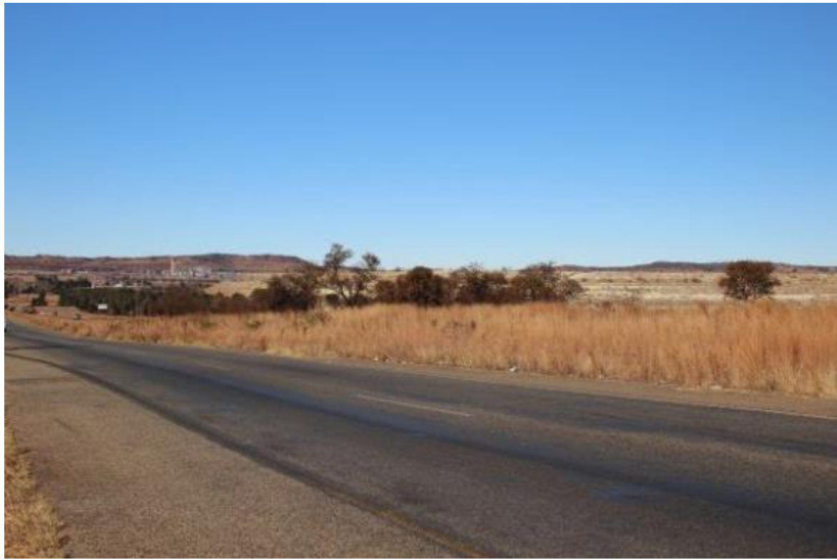
Figure 9: View of Driefontein 5 TSF from the R500 Regional Road
