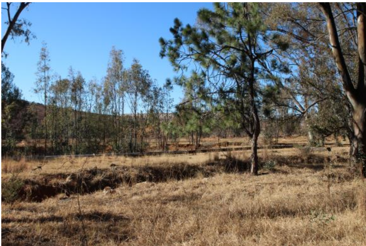
Figure 1: View of Pipeline in the Driefontein MRA from 20 m
