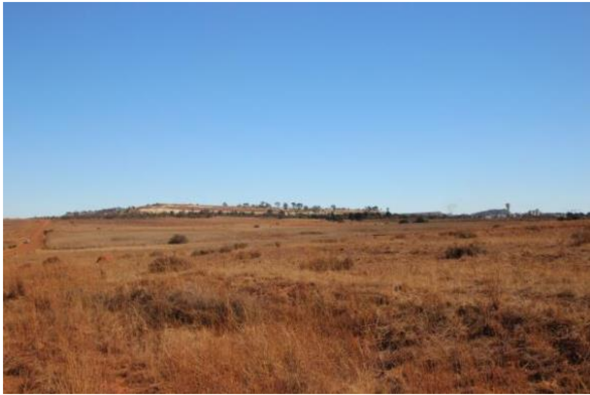
Figure 12: View of Cooke 4 South TSF from Secondary Road
