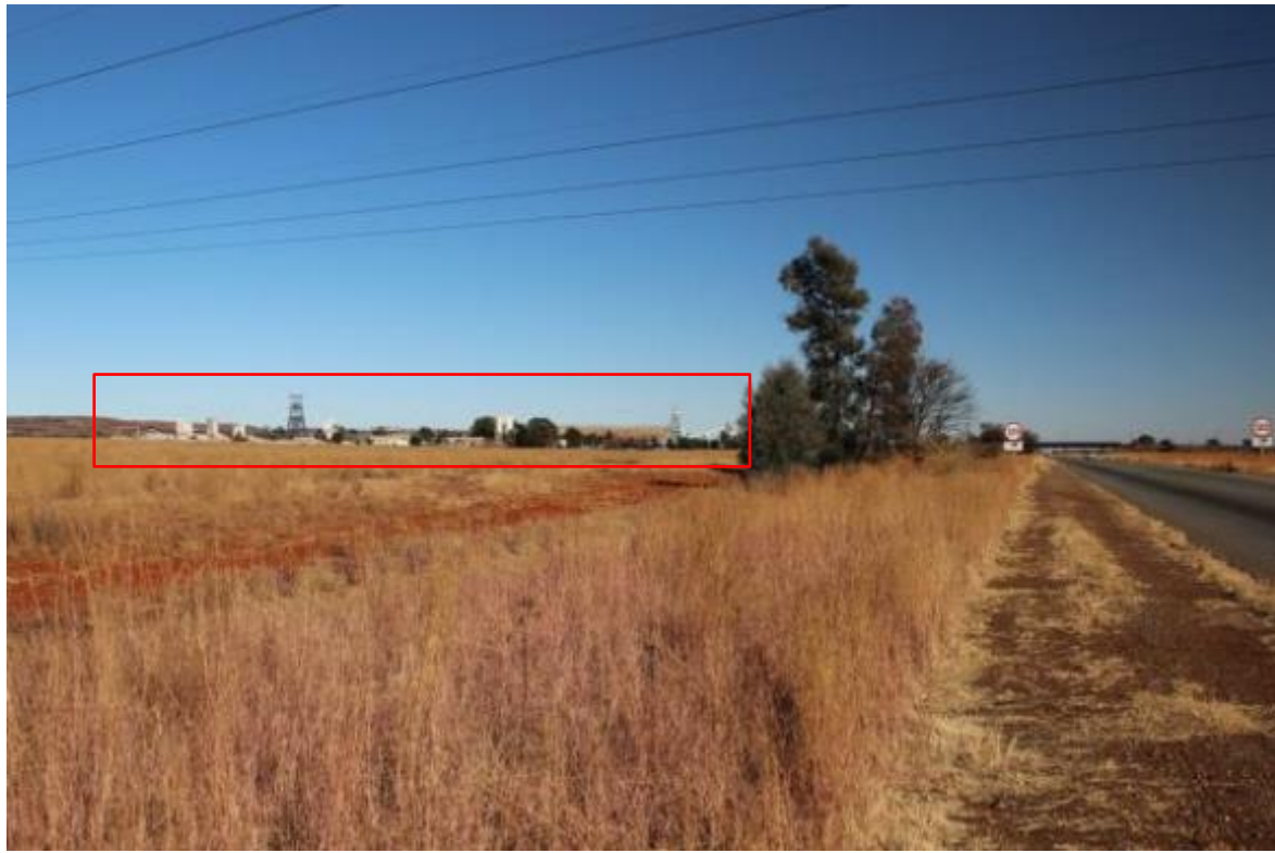
Figure 3: View of Plant Infrastructure in the Driefontein MRA from 0.8 km
