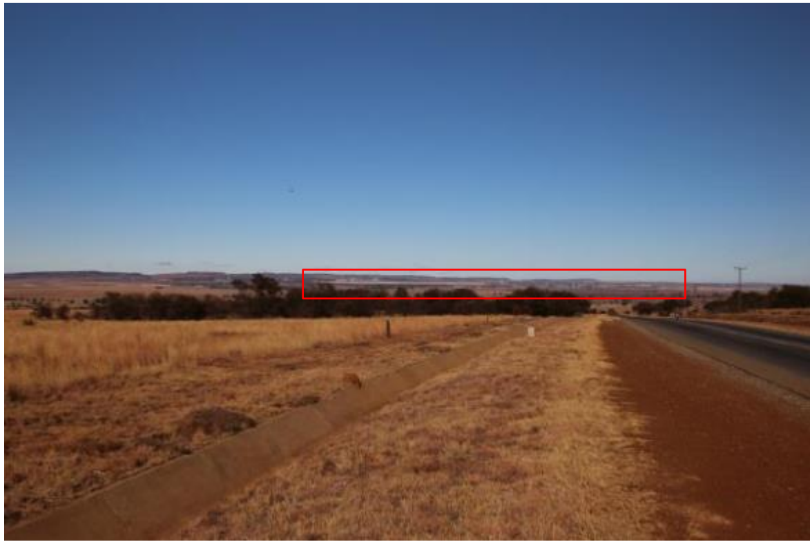
Figure 6: View of Driefontein 1 TSF from 11.4 km, Driefontein 2 TSF from 10.8 km and Driefontein 4 TSF from 12.2 km
