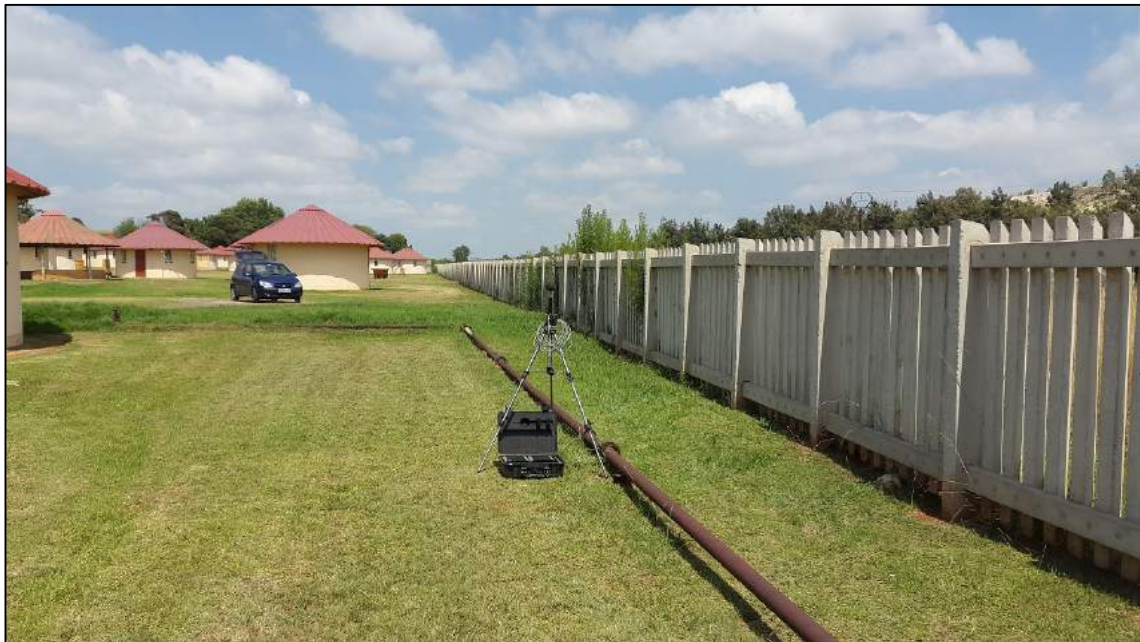
Figure 3: N3 measurement location
