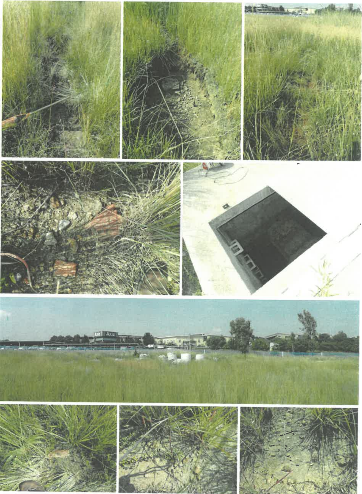
Figure 35 Site conditions, vegetation signatures, infrastructure (pipes) and erosion signatures
