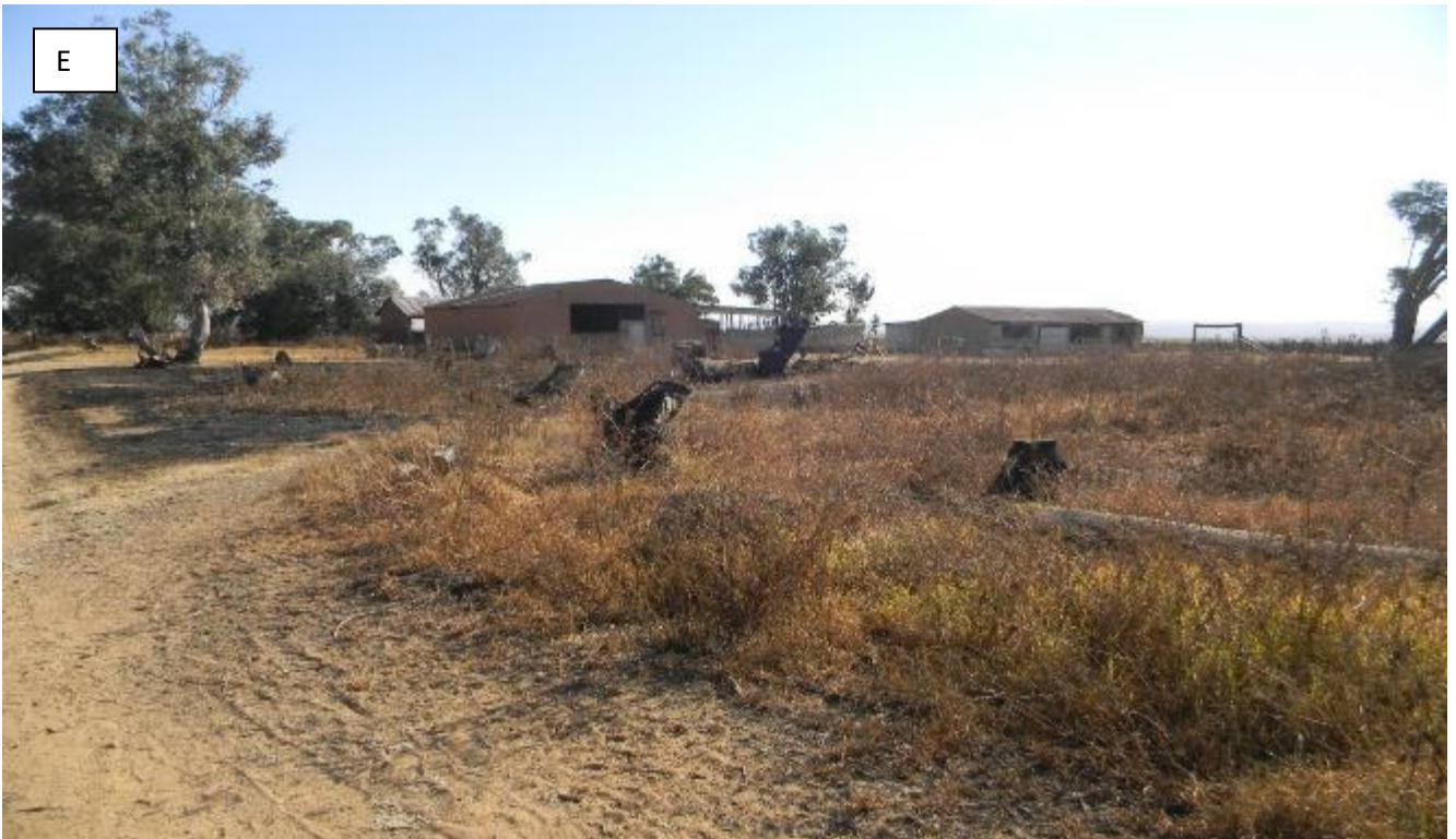
Plate 5: Photo E showing some farm structures associated with historical building.
