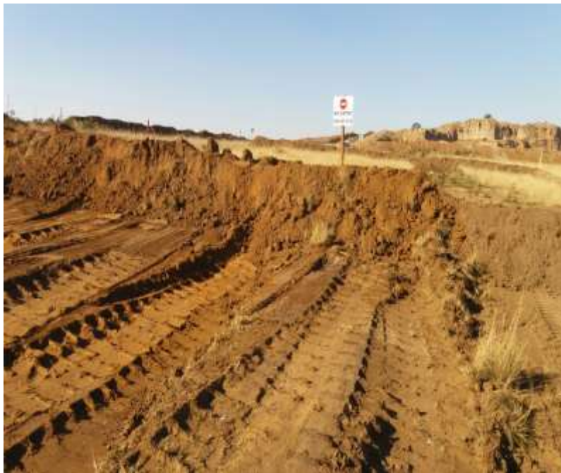
Fig.14: The Warning Signs at Site 2.
