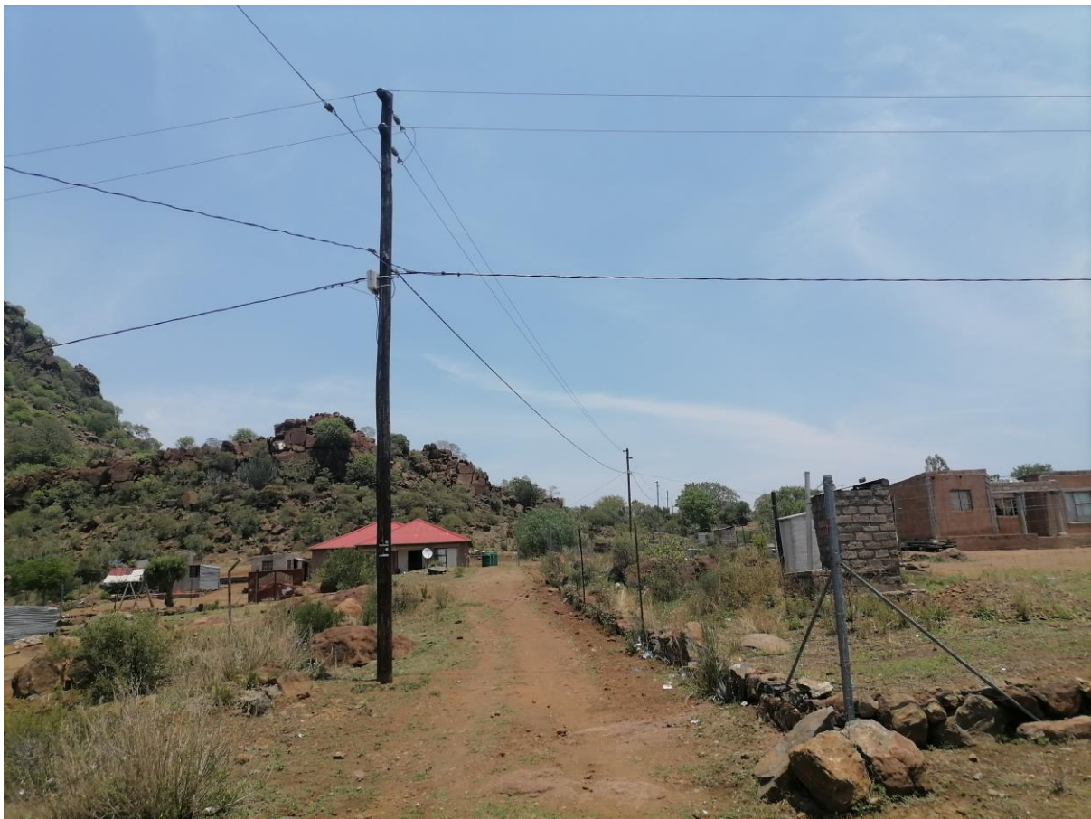
Picture 2: Shows the existing poles in the area and houses
