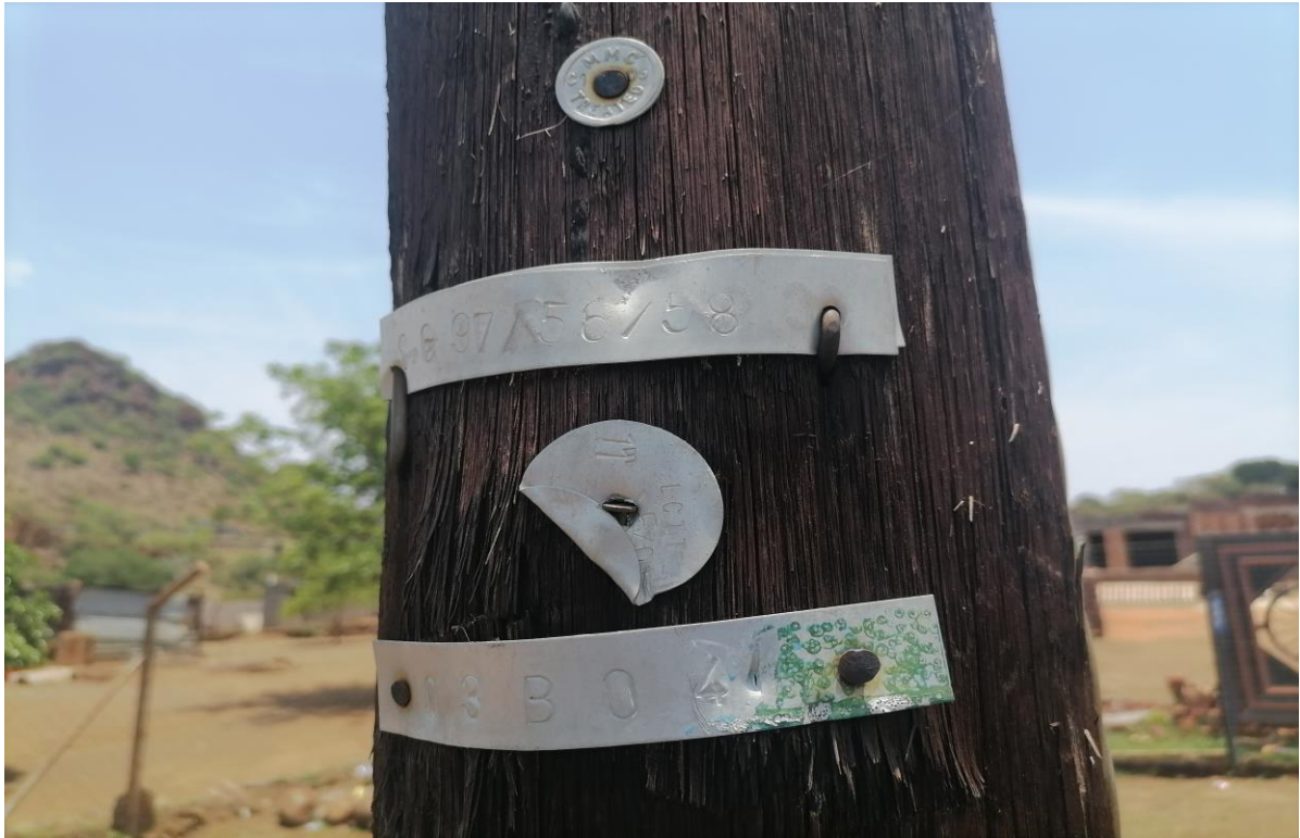
Picture 1: Shows the existing pole number
