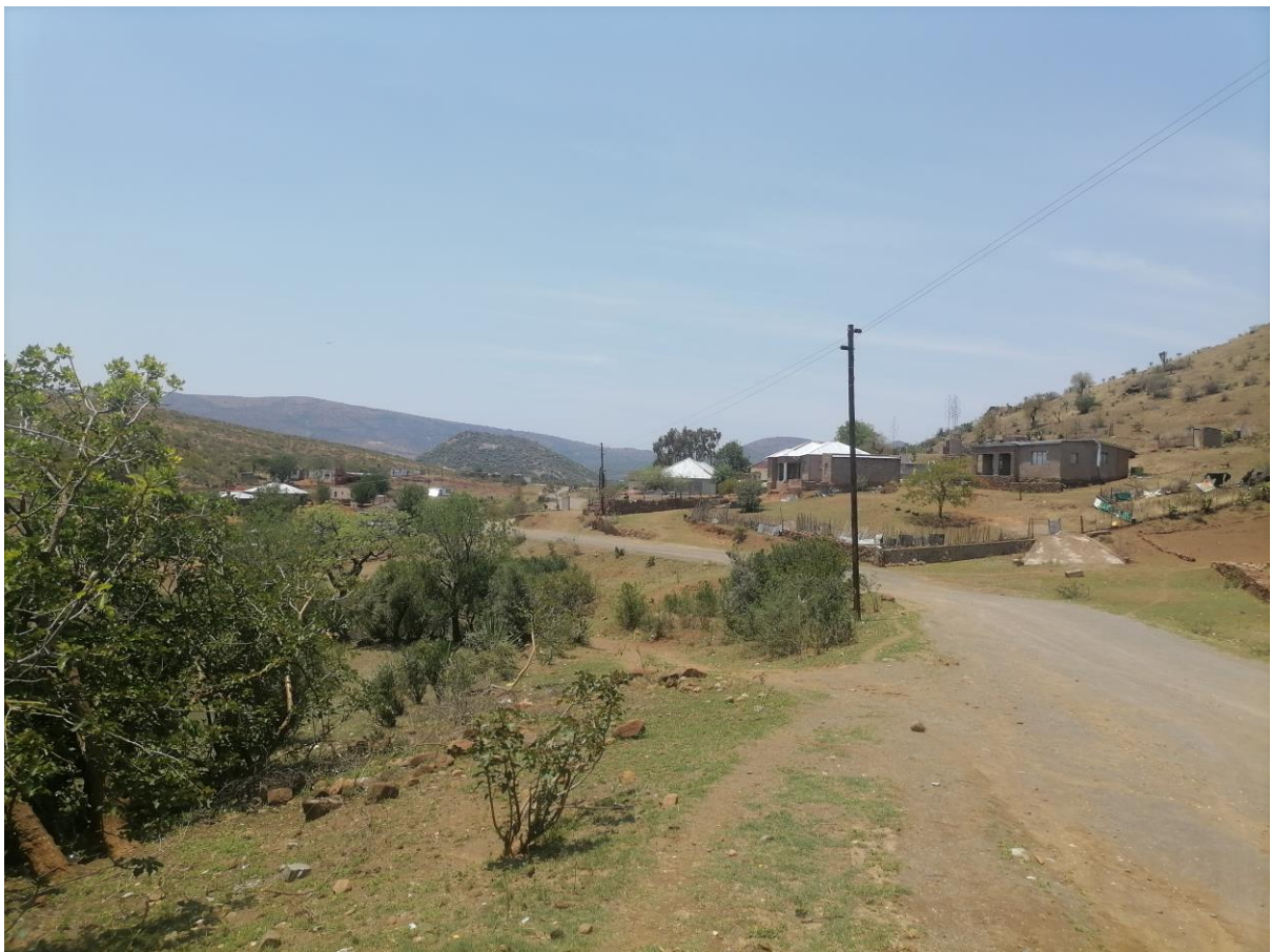
Picture 4: Shows the pole where the line will be deviated and connected
