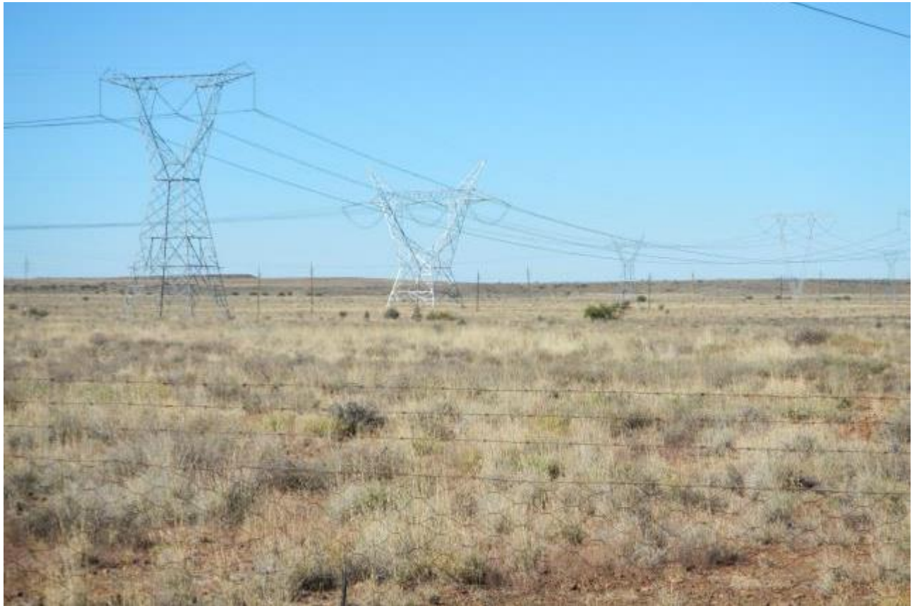
Figure 3: Existing transmission lines near Droërvier Substation
