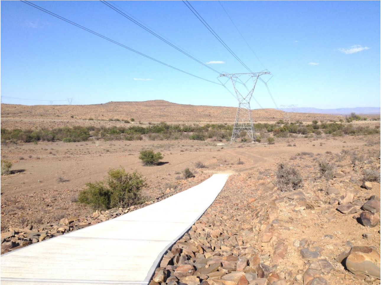
Photo 12 Concrete track below an Eskom line east-east of Merweville.
