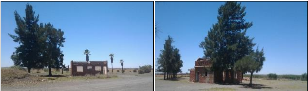
Plate 2.2: Existing buildings to be demolished.
