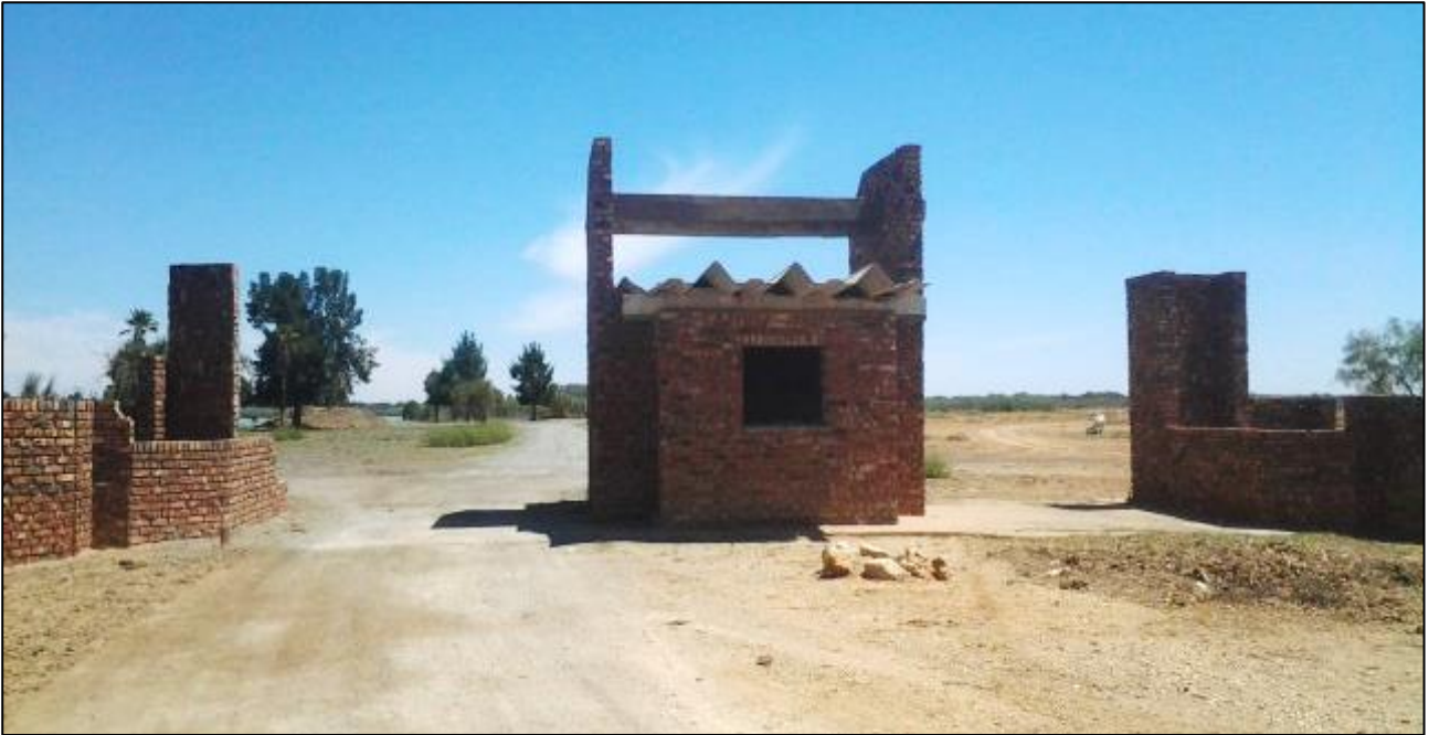
Plate 2.1: Existing entrance: buildings to be demolished and replaced by reception, security and information centre (refer to Fig 7.a).
