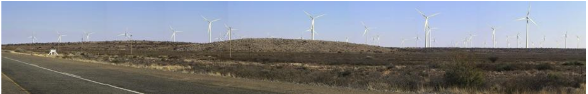
Figure 7.9b: Post construction panoramic overview from view point 1
