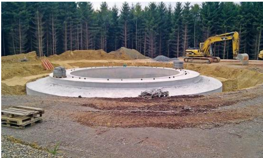
Figure 5.2: Photograph illustrating a completed foundation for a wind turbine (photo sourced from www.juwi.com )
