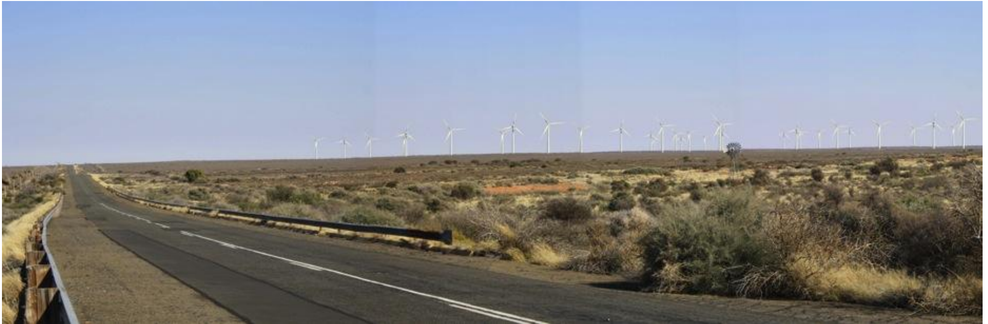
Figure 7.10b: Post construction panoramic overview from view point 2
