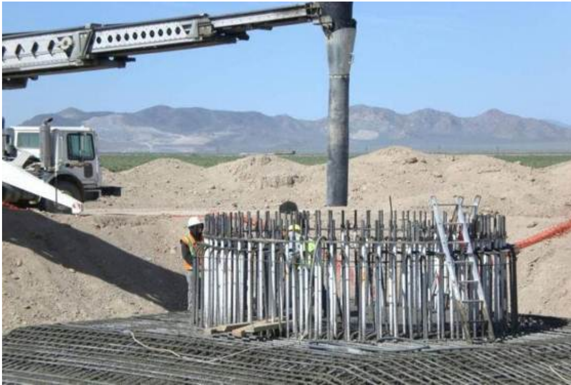
Figure 5.1: Photograph illustrating the construction of the foundation for a wind turbine (photo sourced from www.blm.gov )
