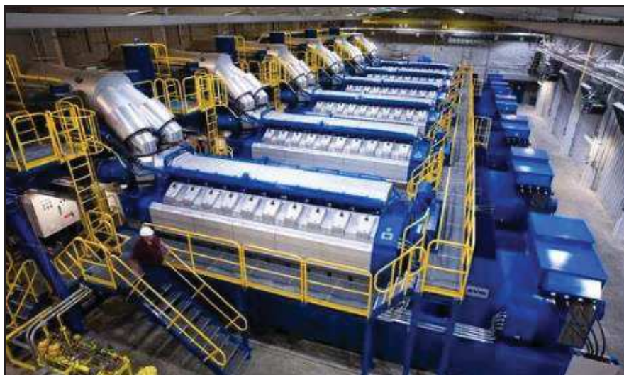
Figure 2-8: Example of a typical Combined Cycle Internal Combustion Engine setup (Source: Wartsila)
