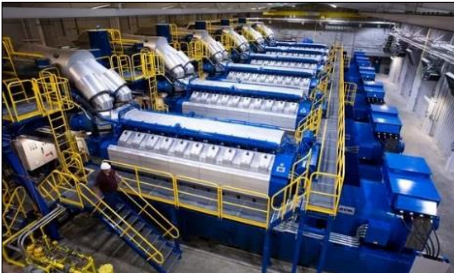
Figure 2-8: Example of a typical Combined Cycle Internal Combustion Engine setup (Source: Wartsila)
