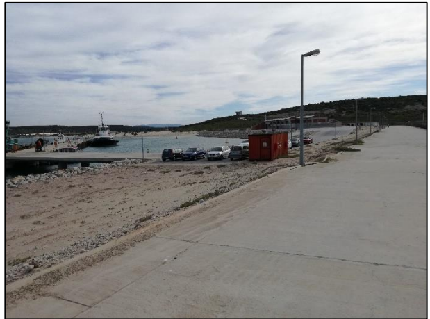
Photograph 6: View northwards along the eastern breakwater showing pipeline alignment
