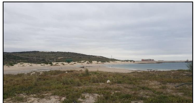
Figure 0-3: Overview of Port Site
