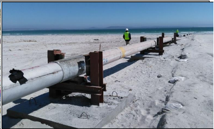
Figure 2-7 Typical Launchway across beach
