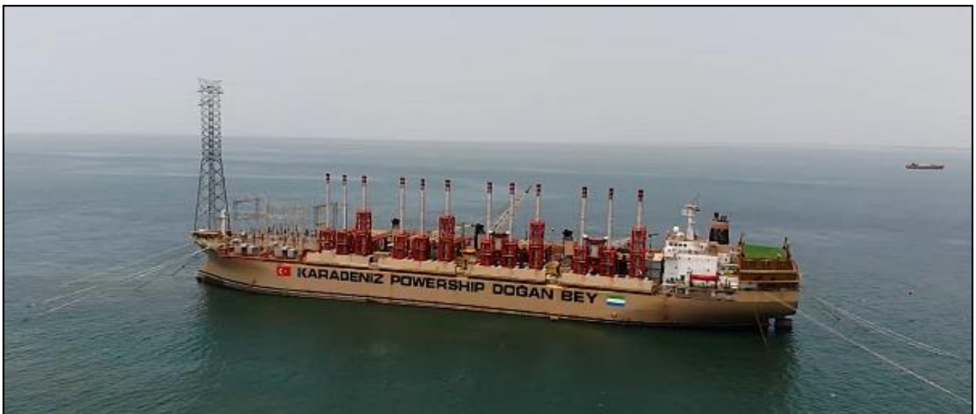
Figure 3-3: Powership mooring system.
