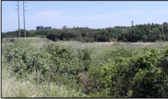
Figure 0-4: Overview of Transmission Route
