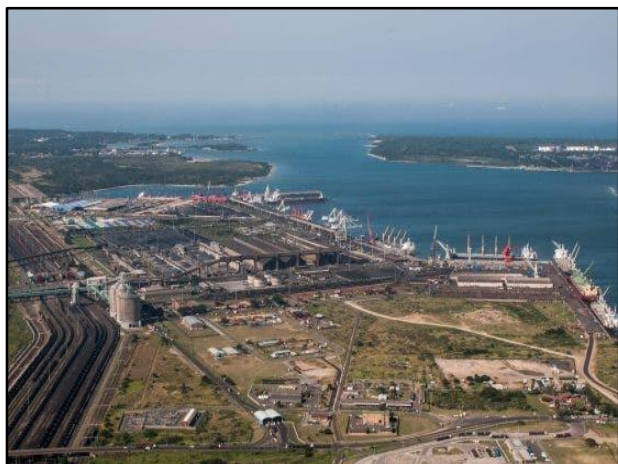
Figure 0-1: Overview of the Port of Richards Bay
