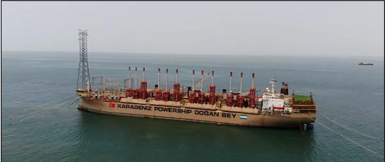
Figure 3-2: Powership mooring system.
