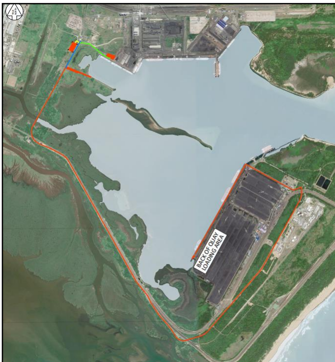
Figure 2-12: Existing access road to the proposed load-out berth
