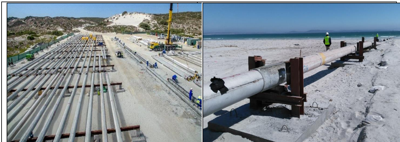
Figure 2-7: Typical Stringing Yard
