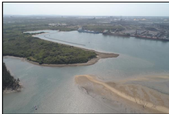
Figure 0-3: Overview of Port Site
