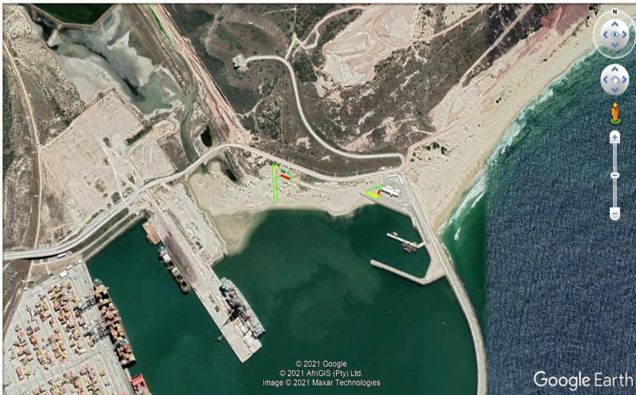
Figure 9-2: Proposed location for the temporary laydown area for the installation of the gas pipeline.
