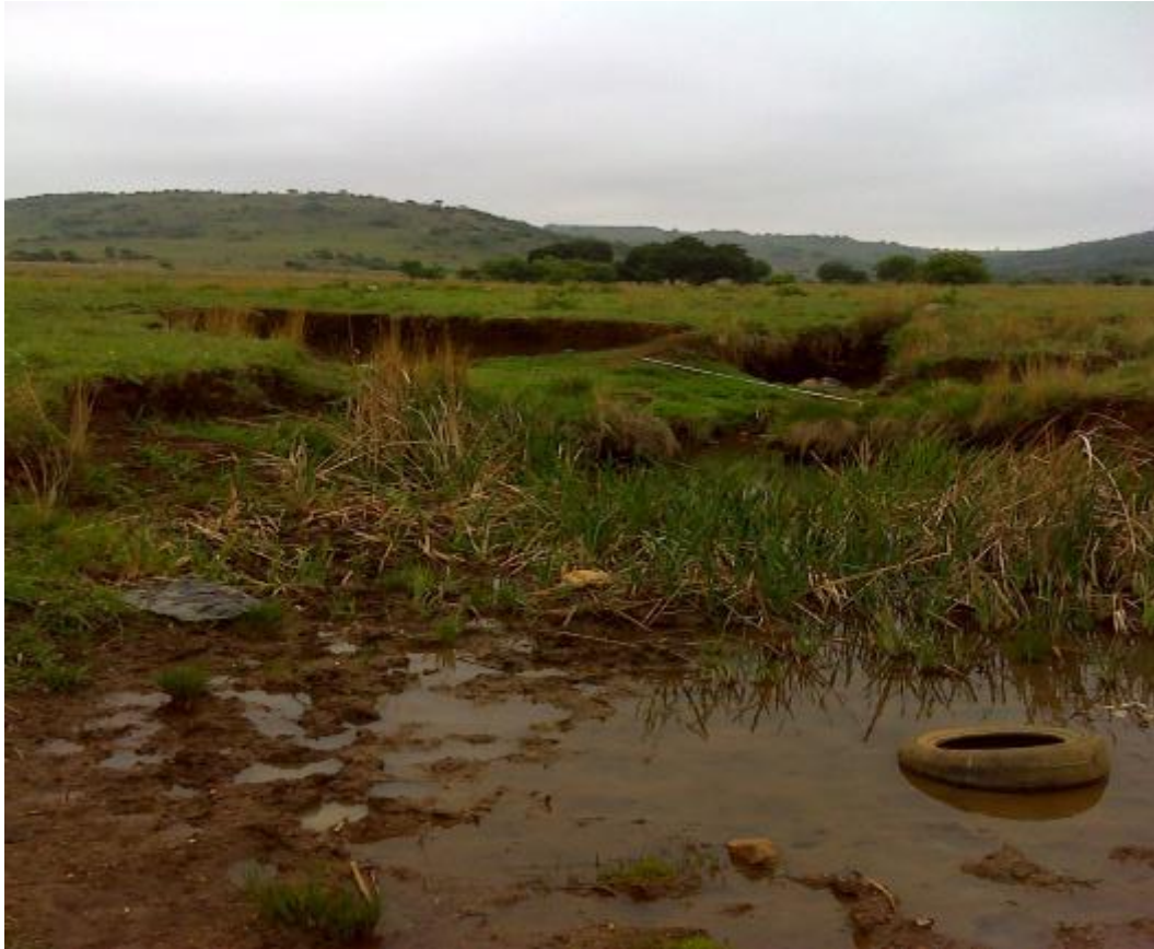
Figure 9: Photograph indication active multiple headcut to be monitored on site post rehabilitation
