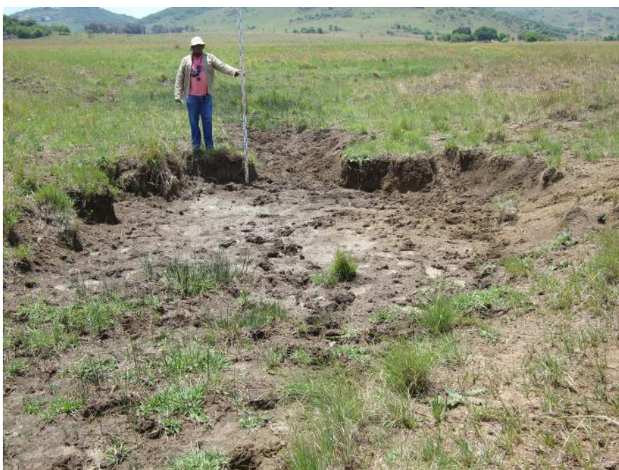
Figure 19: Photo of intervention site C22D-04-209-00
