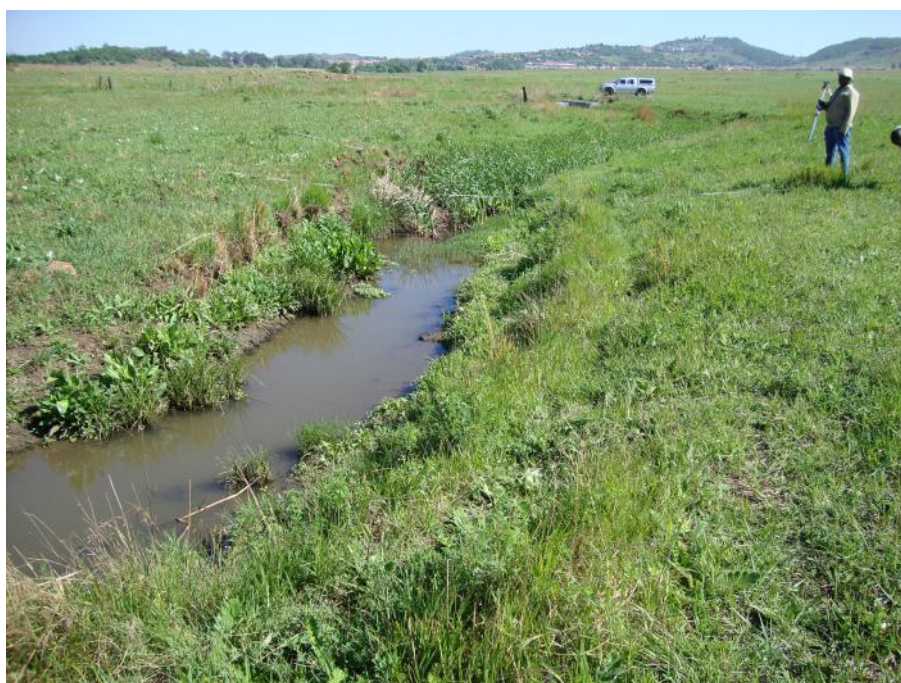
Figure 23: Photo of intervention site C22D-04-213-00
