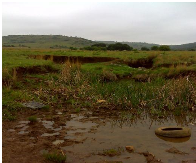
Figure 26: Photograph indication active multiple headcut to be monitored on site post rehabilitation
