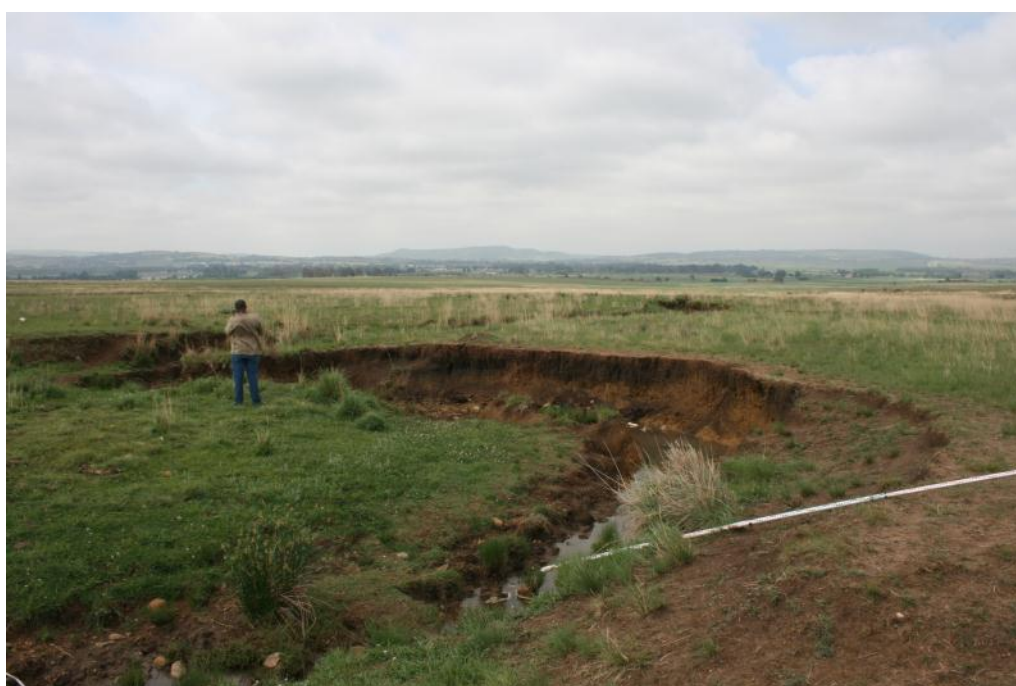
Figure 14: Photo of intervention site C22D-04-204-00
