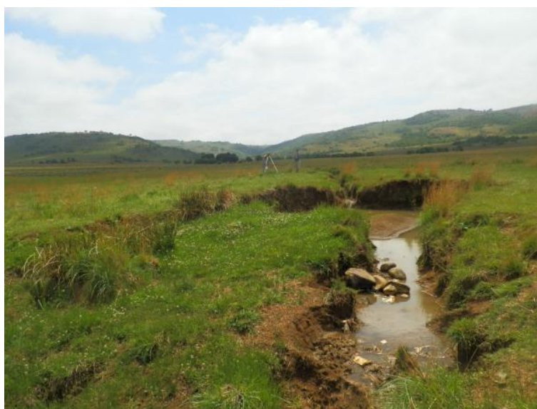
Figure 27: Photograph indication active headcut erosion to be monitored post rehabilitation on site.
