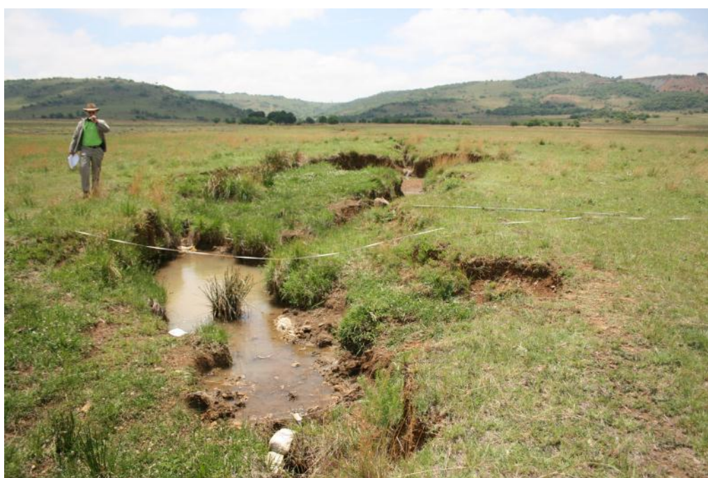
Figure 18: Photo of intervention site C22D-04-208-00
