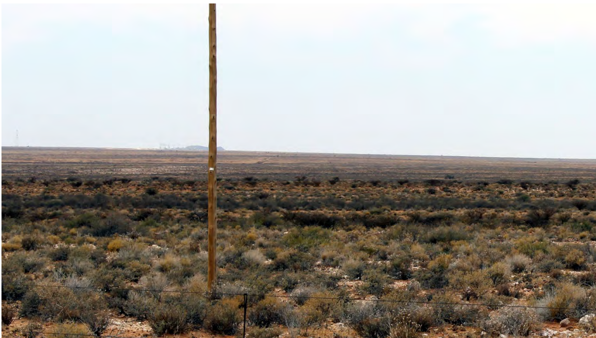
Figure 7-15 View from photo site SCA014 eastwards. The tower at Rugseer Siding is visible on the left and the new substation more towards the centre.
