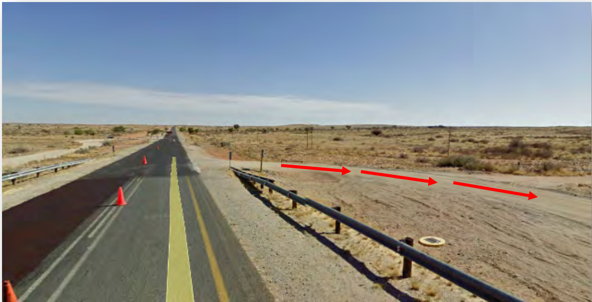
Photo 16.3: The intersection of the R27 and Transnet Service Road, going towards Keimoes (Image source: Google, 2010)
