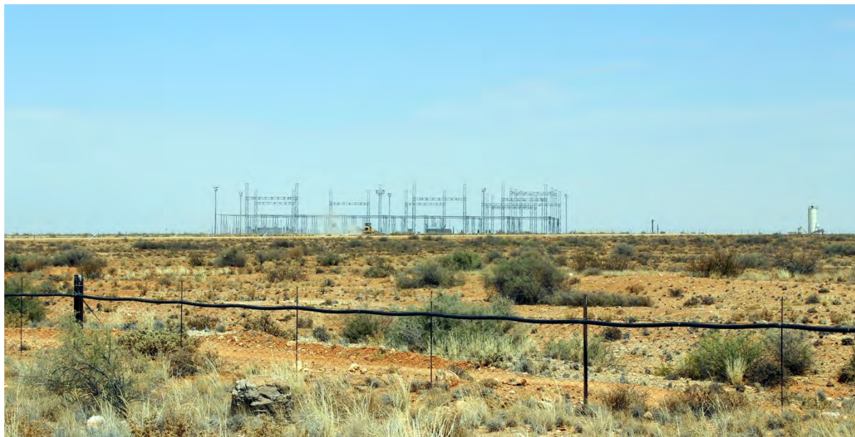
Figure 7-16 Nieuwehoop Substation currently under construction (Photo site SCA010)
