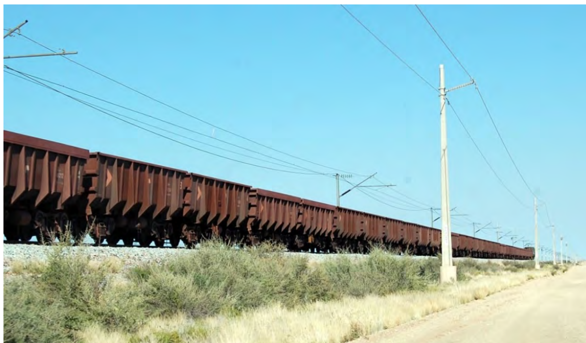
Figure 7-13 Empty ore train on the Saldanha-Sishen railway line.
