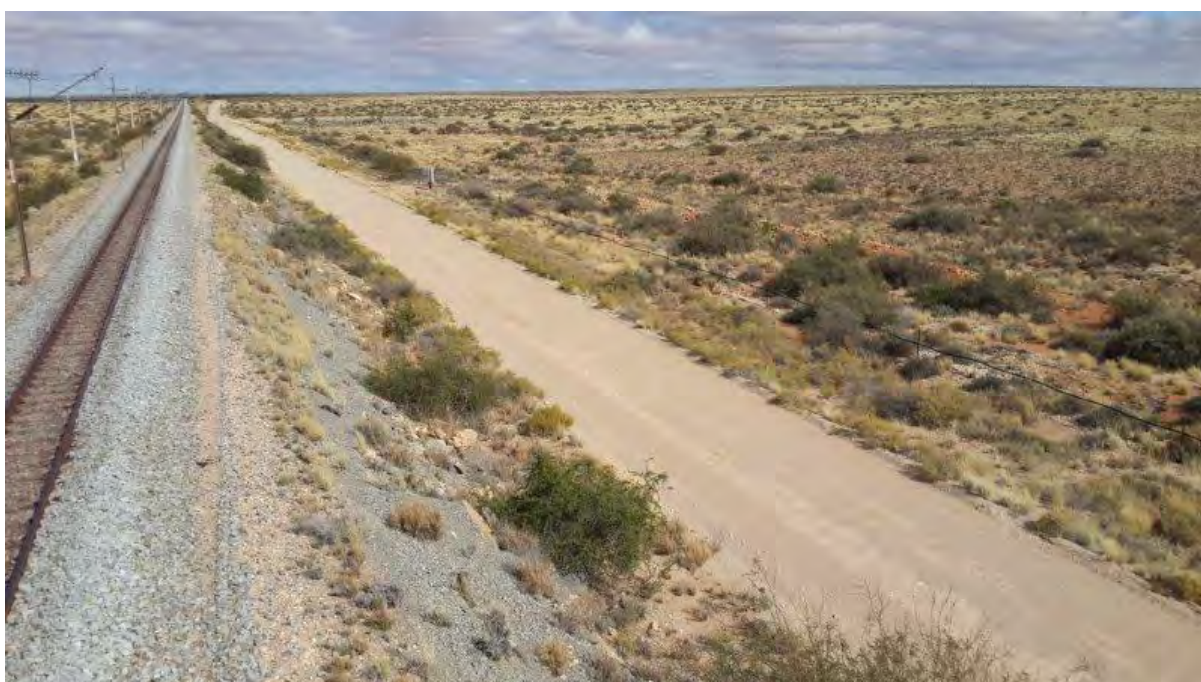
Figure 11.4: Photograph showing the railway and road running through the farm and the typical site conditions.
