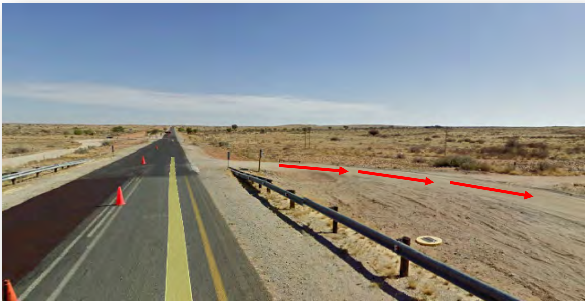
Photo 16.3: The intersection of the R27 and Transnet Service Road, going towards Keimoes (Image source: Google, 2010)
