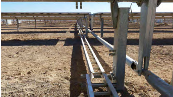
Figure 35: Proposed single axis tracking system to be used for the proposed Mulilo PV projects.
