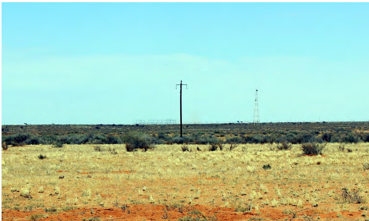
Figure 7-14 The tower at the Rugseer Siding as seen from photo site SCA011..
