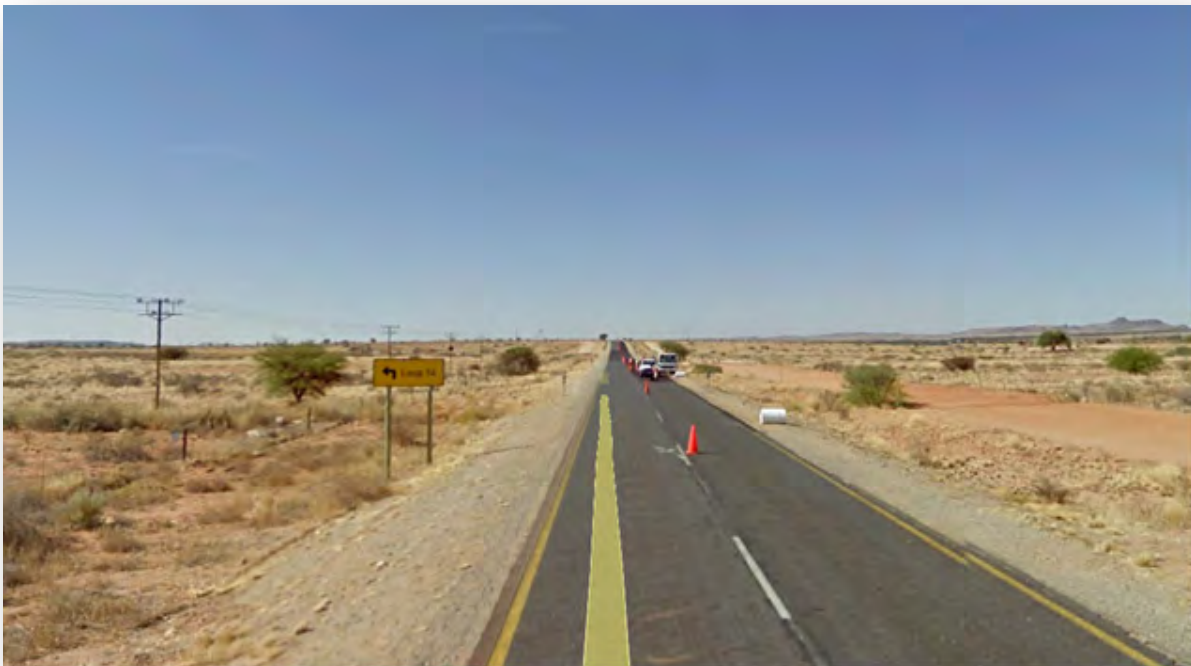
Photo 16.1: R27 towards the south (taken towards Kenhardt). The board shows “Loop 14”, located to the left, which is accessed via the Transnet Service Road. (Image source: Google, 2010)
