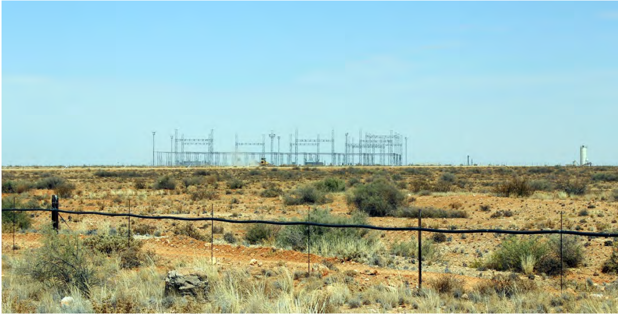
Figure 7-16 Nieuwehoop Substation currently under construction (Photo site SCA010)
