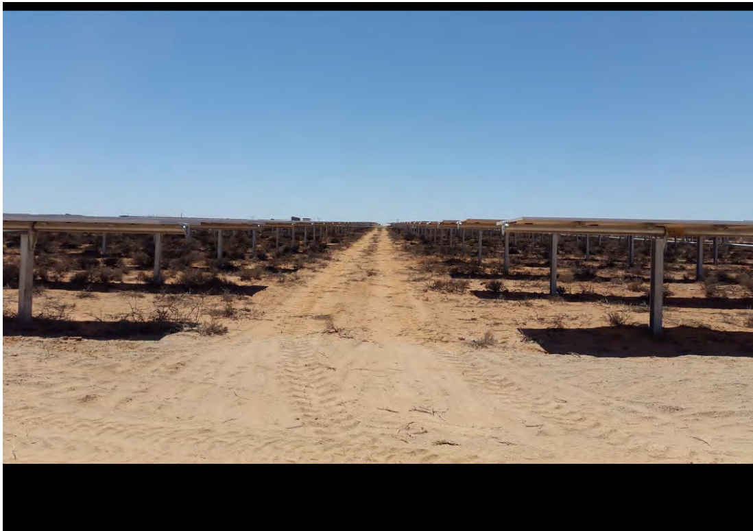
Figure 2.7: The vegetation underneath the solar panels will not be cleared, but will remain intact (Source: Mulilo Renewable Project Developments)
