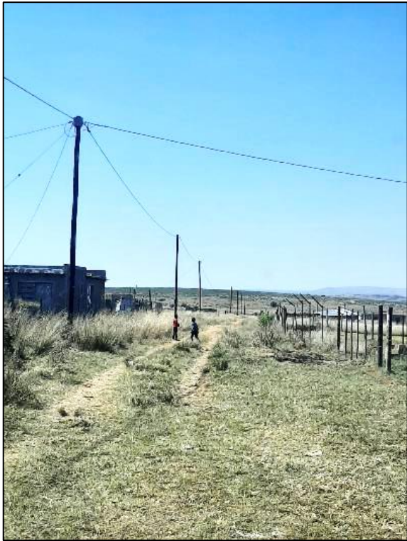
Images 7: Existing Low Voltage Aerial Bundled Conductor & Airdac reticulation networks
