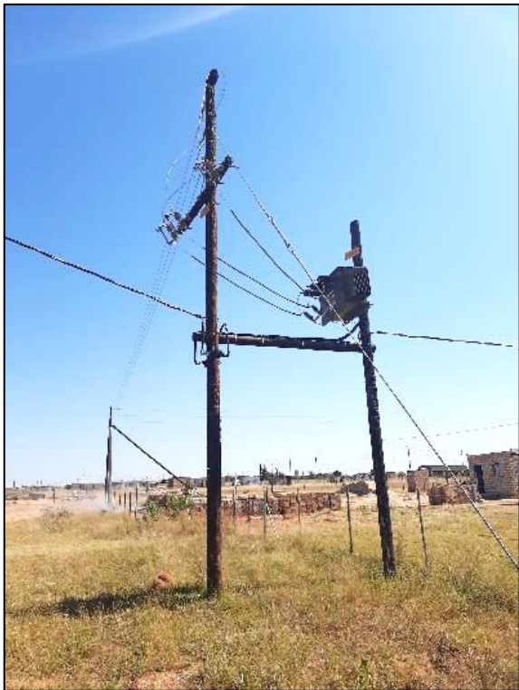
Images 6: Typical pole mounted, 22kV/231V transformers
