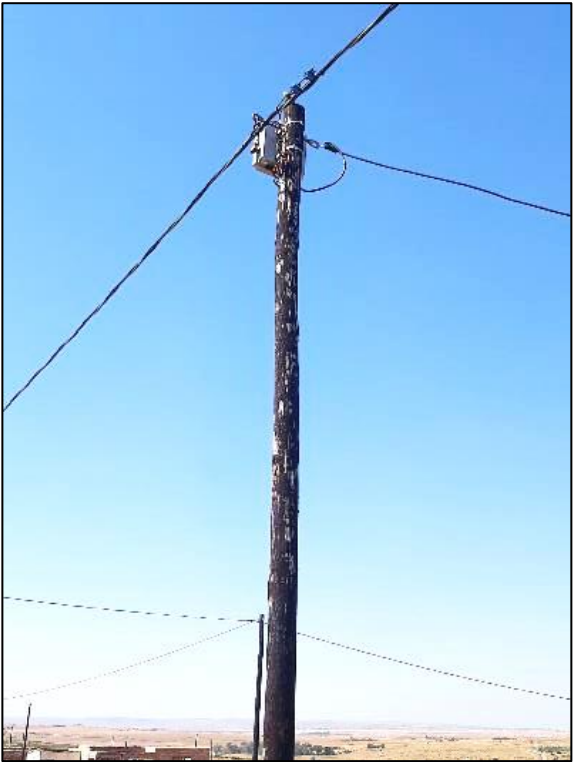
Images 7: Existing Low Voltage Aerial Bundled Conductor & Airdac reticulation networks
