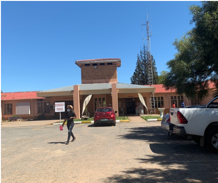
5. View of Existing Hospital Building Entrance
