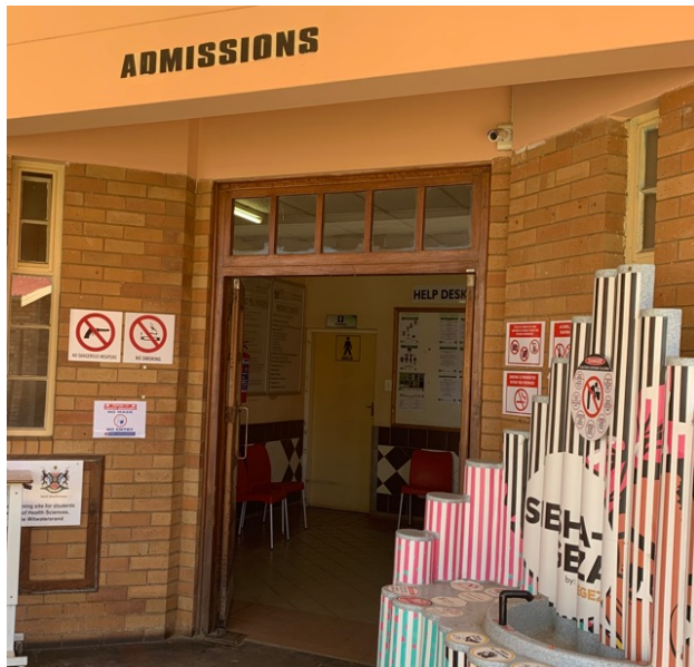
7. View of Existing Hospital Admissions Entrance
