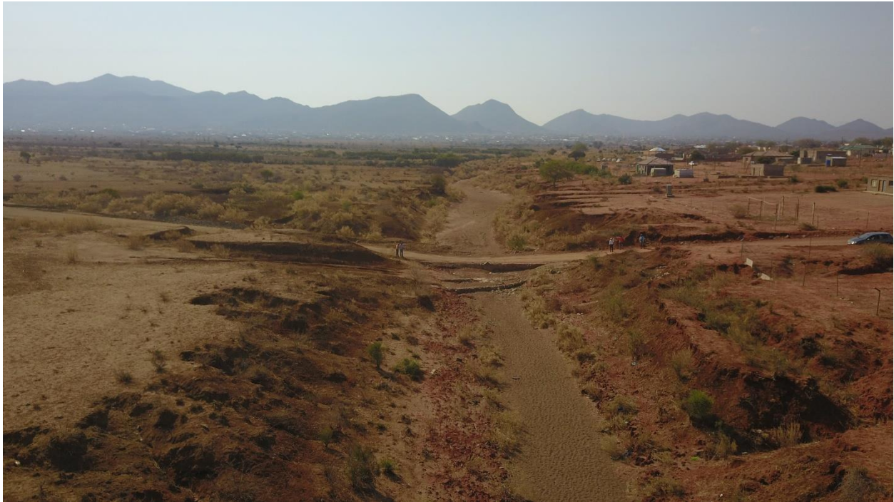
Figure 2-4: Sideways view of the existing stream crossing.
