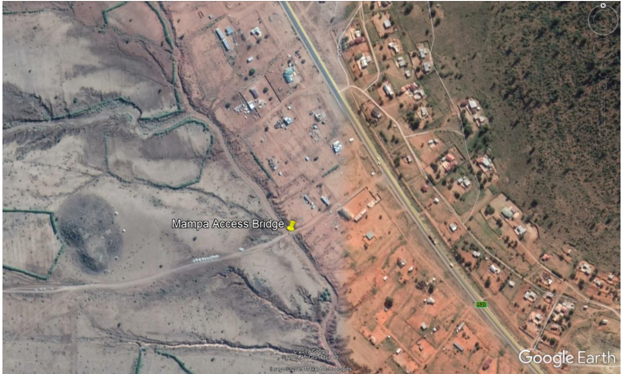
Figure 2-2: Close-up aerial view of Mampa Access Bridge next to R37.
