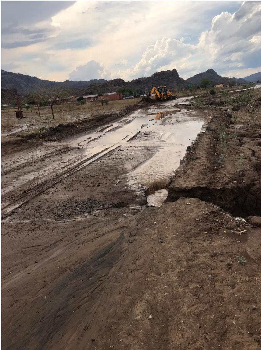
Figure D-3: Condition of Swazi Mnyamane stream crossing at the time of the investigation.
