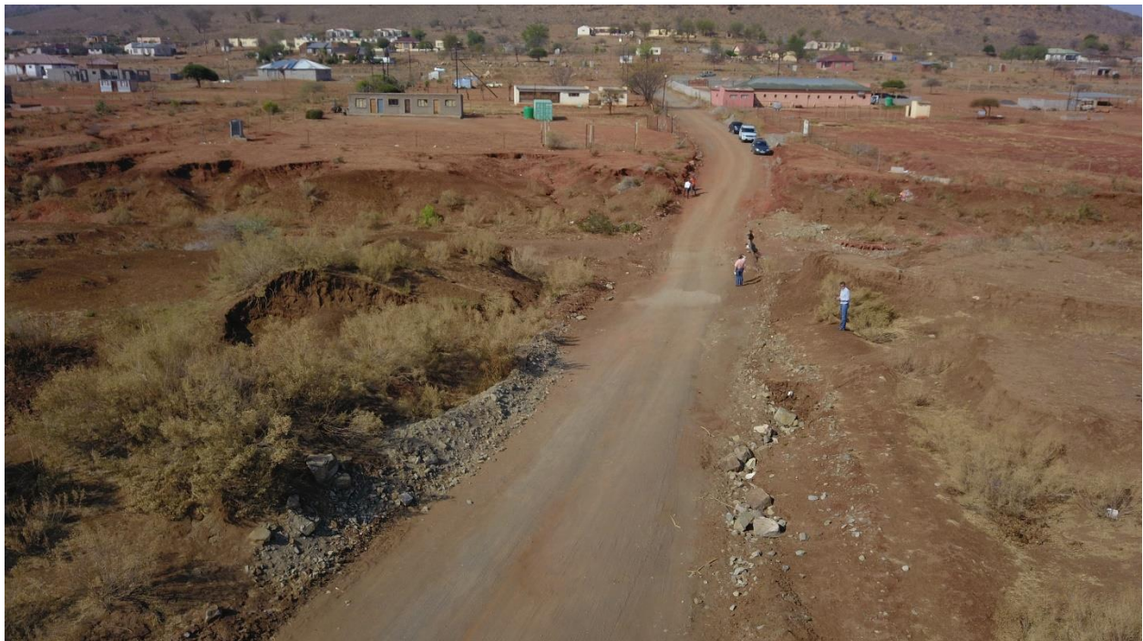
Figure 2-3: View of the existing stream crossing.
