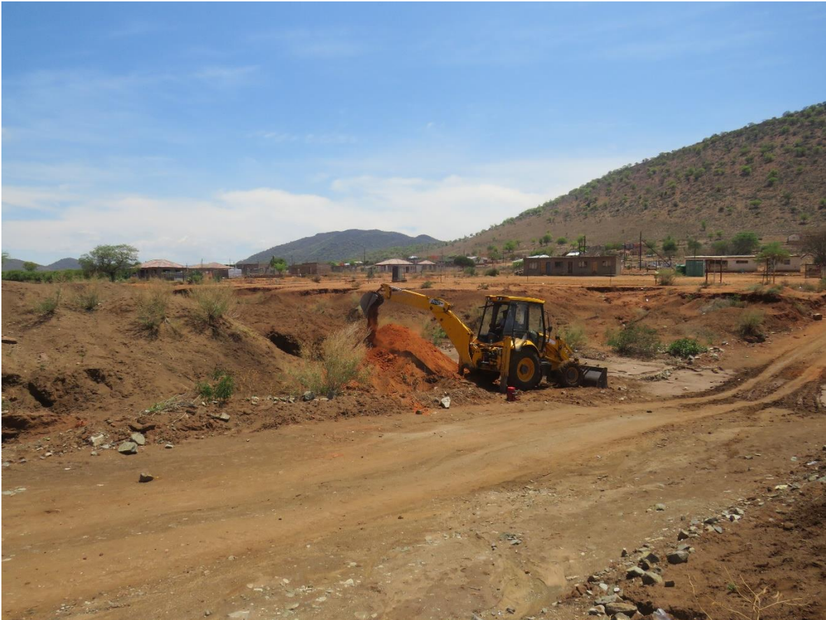
Figure D-1: Excavation of TP-MP01
