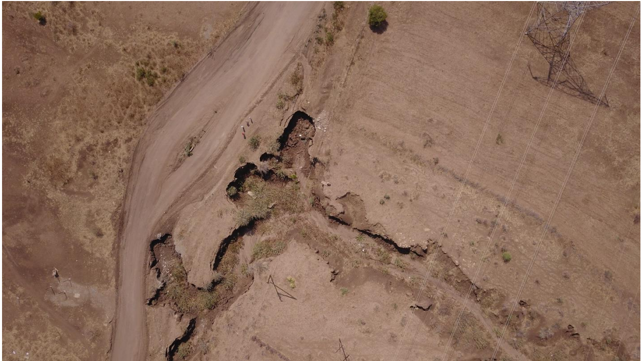
Figure 3-2: View of the existing stream crossing with severe erosion visible downstream (east).
