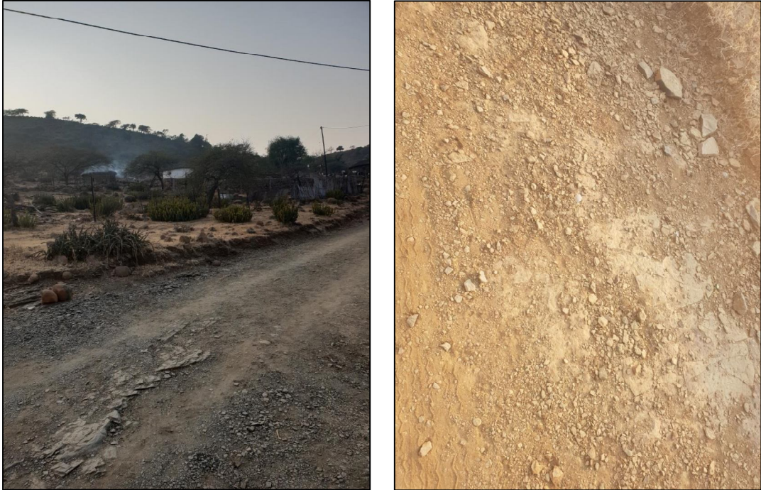
Figure 4&5: Existing road surface, typical of the areas underlain by shale along the proposed route.
