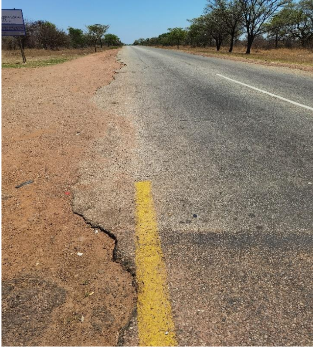
Km 2.95 – km 3.80(Damaged Base)
