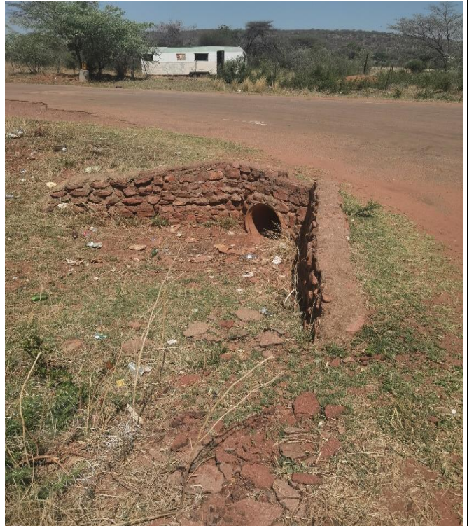
Km 10.13 – Km 11.45 (Existing Culverts )
