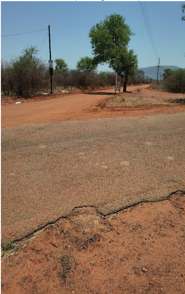
Km 2.95 – km 3.80(Damaged Base)
