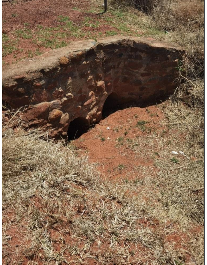
Km 3.8- Km 6.25 (Existing Culvert Structure)
