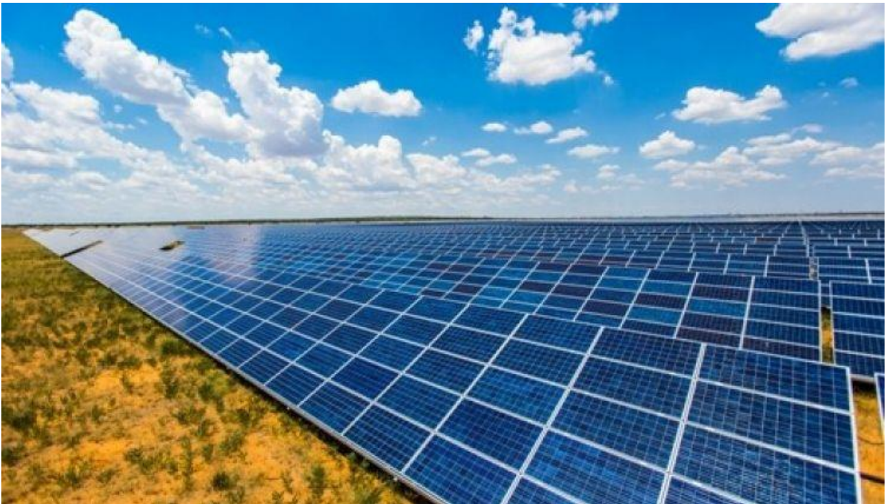
Figure 1: Example of PV Solar Facility (Source: www.pv-tech.org ).
