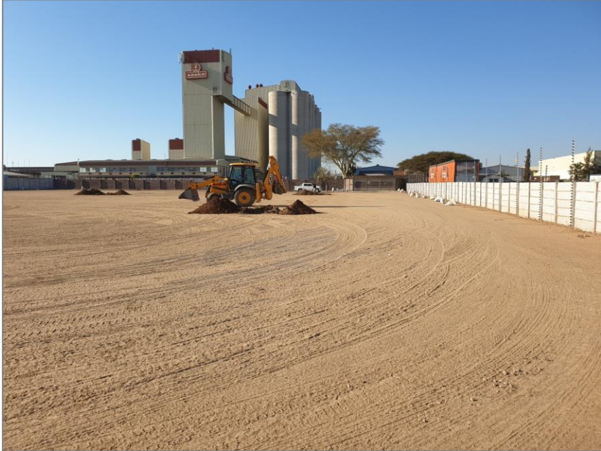
Site Scenery - Test Pit no: TP02
