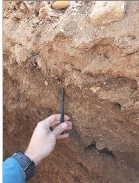
Note: Upper engineered fill material.
