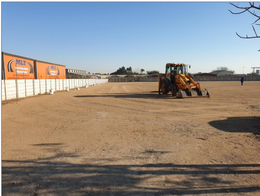
Site Scenery - Test Pit no: TP01
