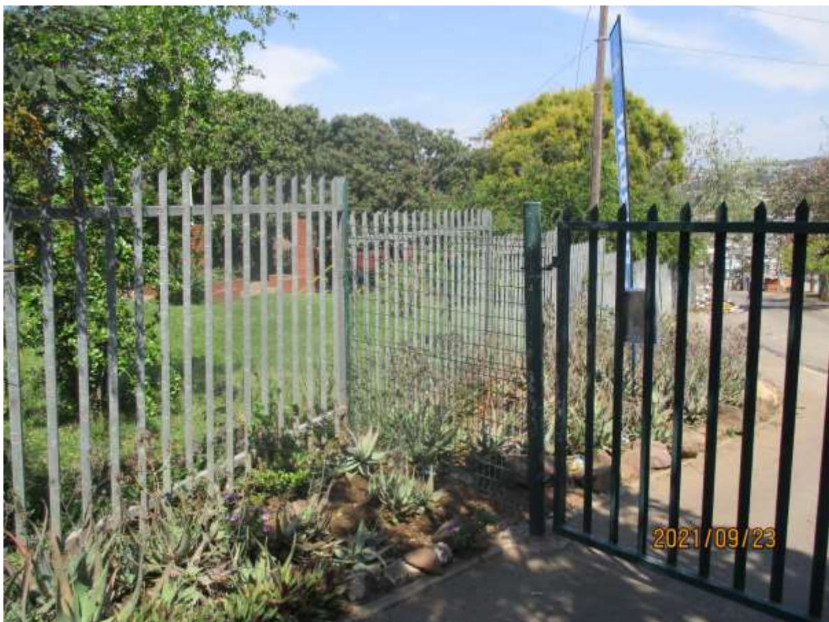
Figure 4: 1,8m Existing Fence (Part palisade, part plasticated mesh)
