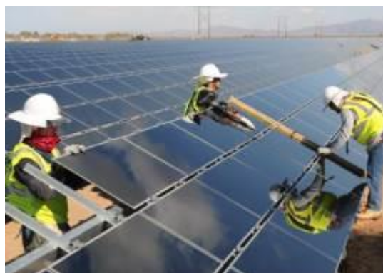
Figure 2.3: Picture of the installation of a typical PV array
