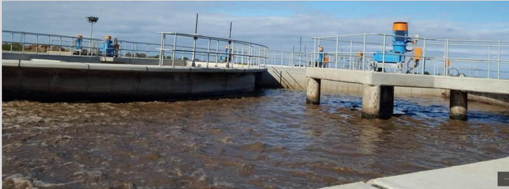
**Figure 7: Aeration zone in the outer channel**
