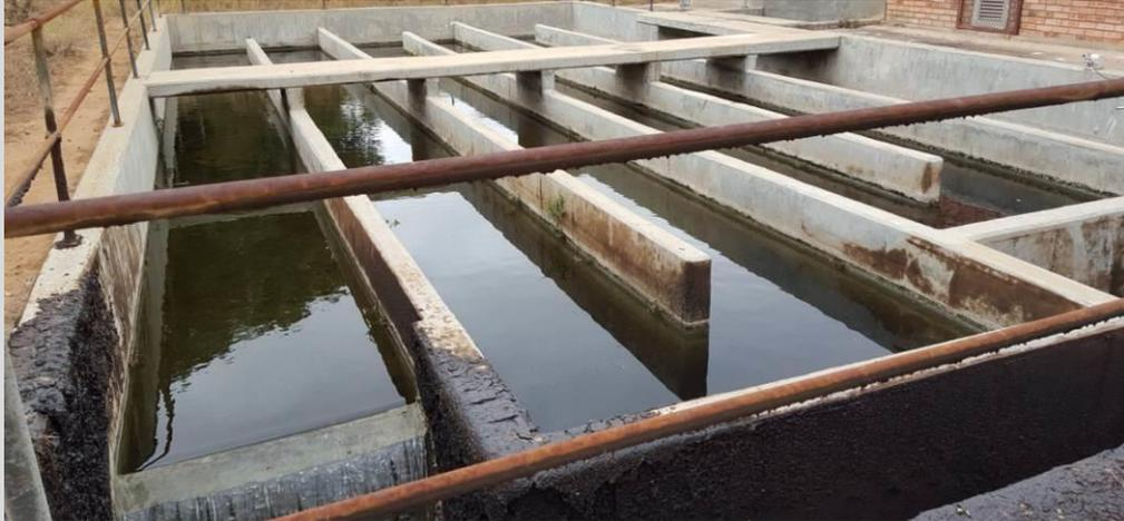
Figure 9: Existing chlorine contact channels
