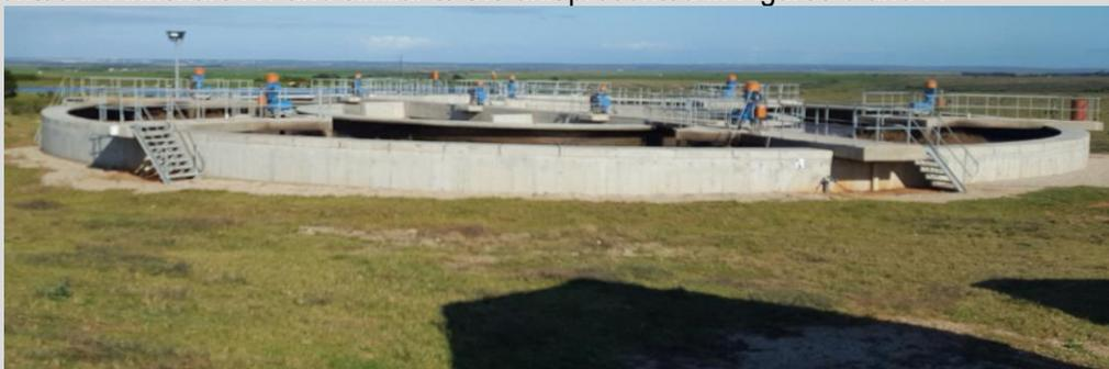
**Figure 6: Typical biological reactor to be constructed**
