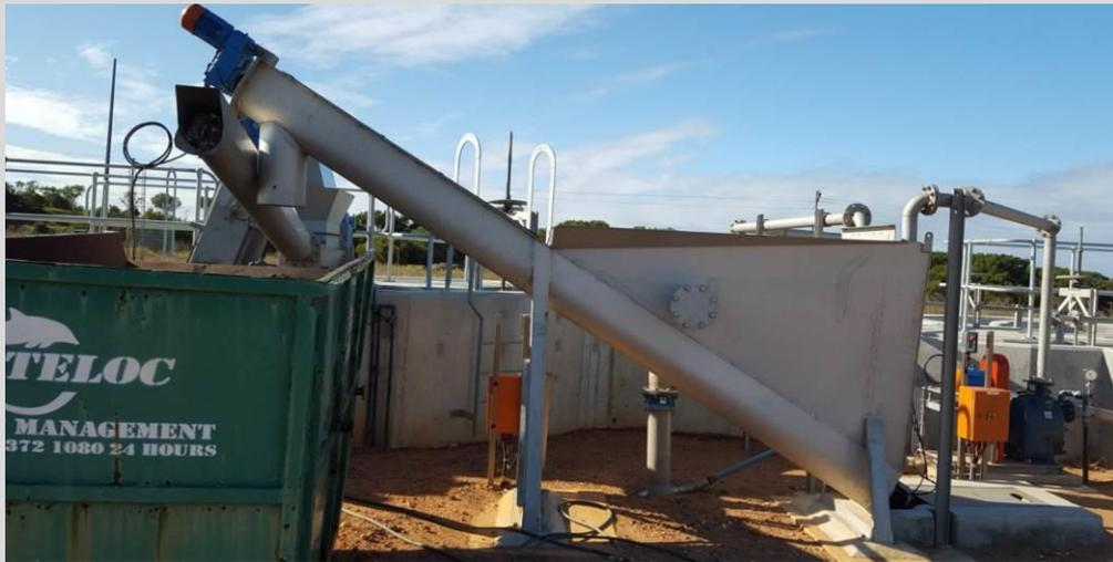
**Figure 5: Mechanical grit conveying into a skip**
