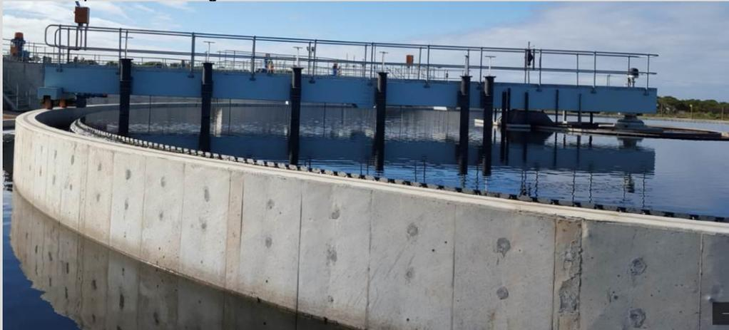
**Figure 8: Typical configuration of the proposed clarifiers**
