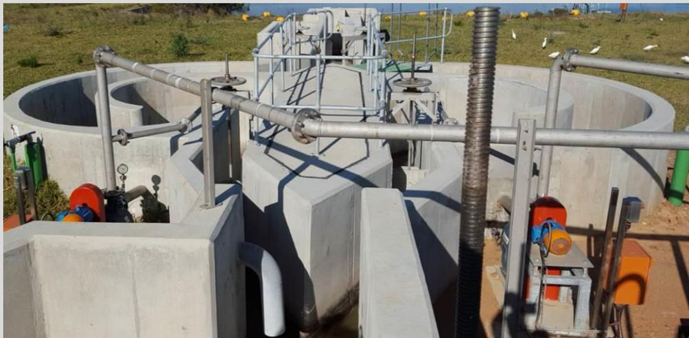
**Figure 4: Two parallel Vortex grit removal mechanisms**
