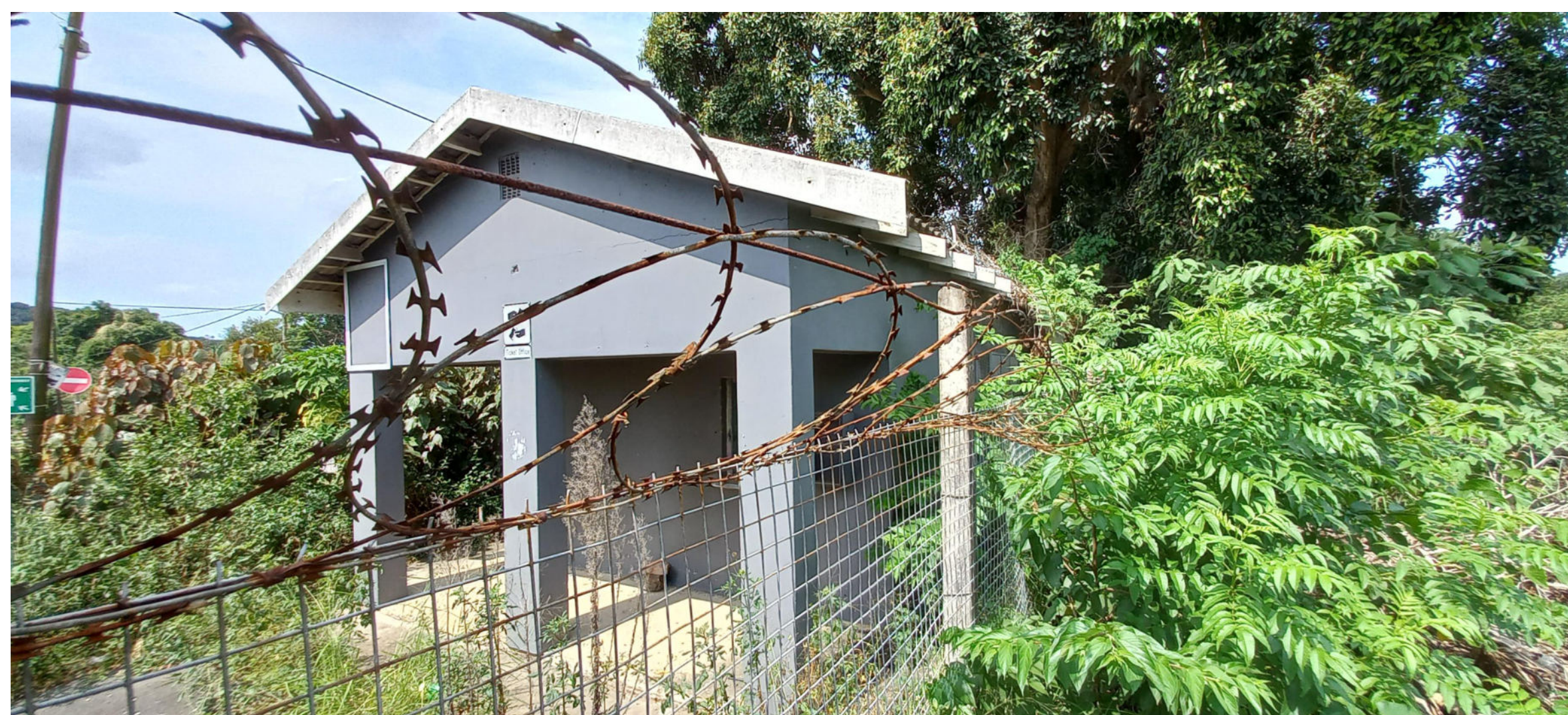
1 - EXISTING TICKET OFFICE
