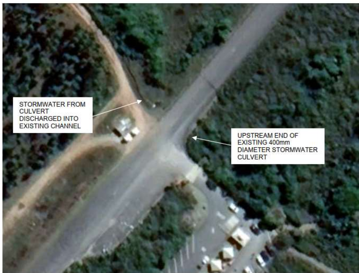
Figure 4-8: Existing stormwater infrastructure
