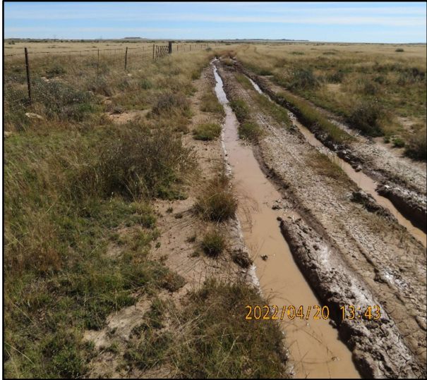
Photo 6: Surface runoff filled farm track along low-lying eastern bank of Brak River (proposed alternative access route crossing from staging area) terrain.
