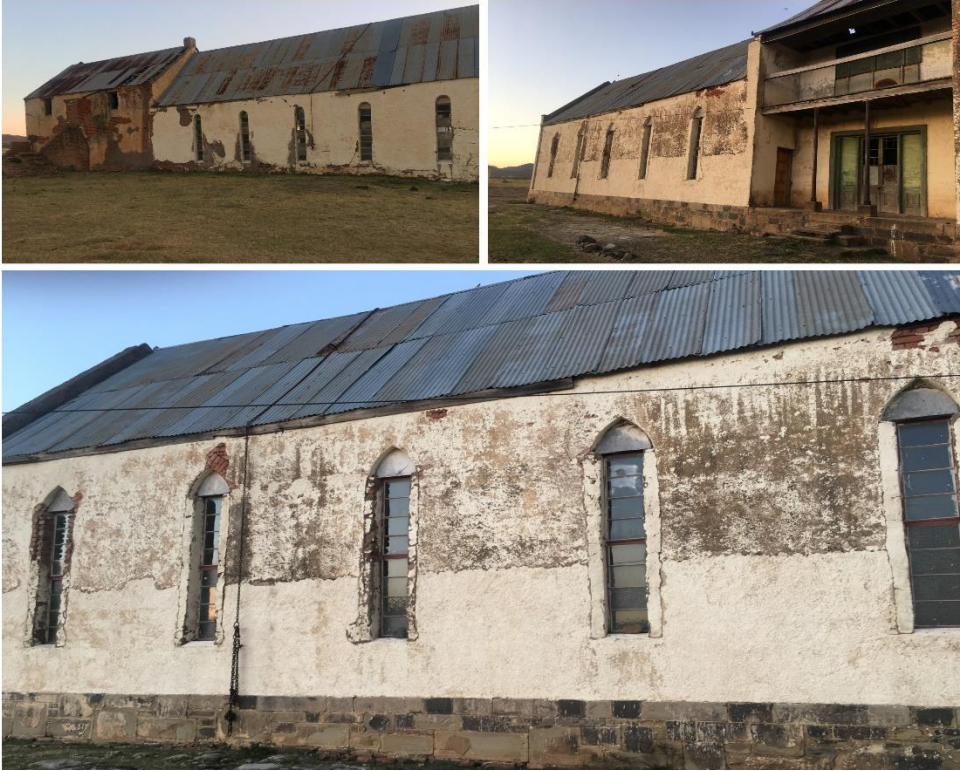
Figure 3: Condition of Church
