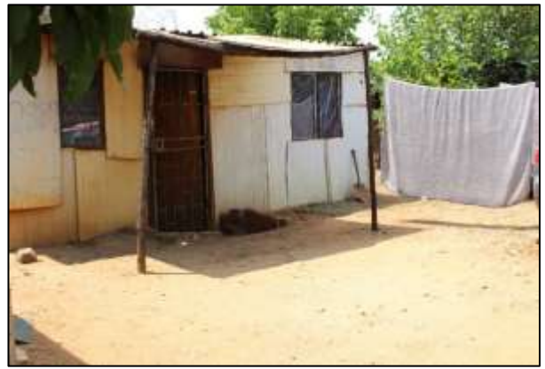
Fig.4 The informal structure built inside the enclosure where graves are located.
