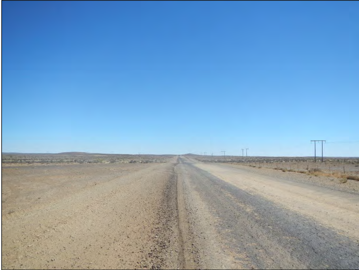
Figure 21: View of the district road that connects the town of Loeriesfontein with Granaatboskolk to the north. This district road is however found well outside the visual impact zone.
