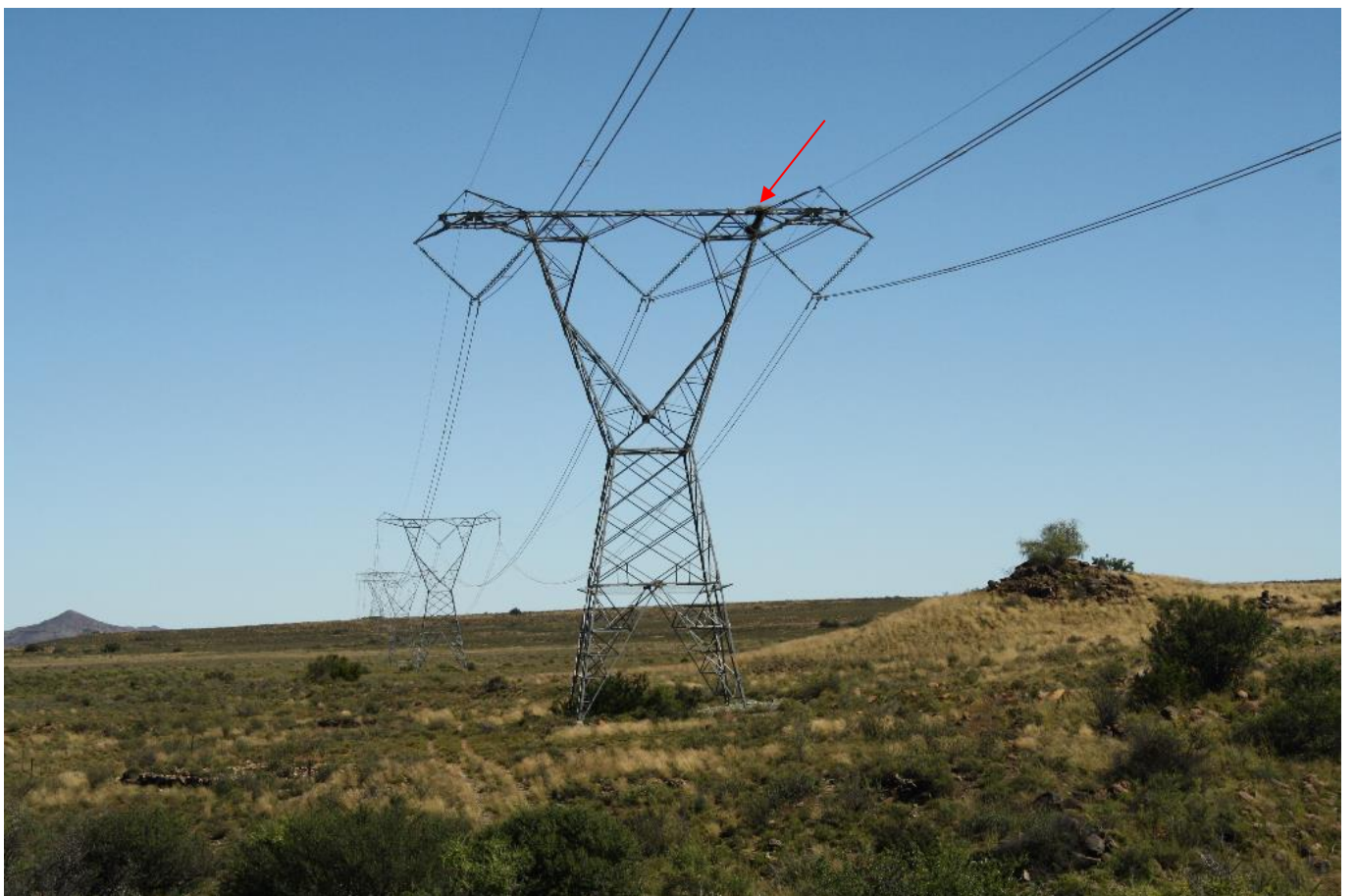
Figure 6: Existing Droërvier Hydra 400kV transmission power line with Tawny Eagle nest in the study area (shown is the red arrow)
