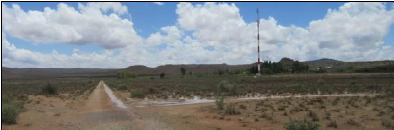
Photograph 3.7: Cell phone relay tower on Bultfontein seen from the N1.
