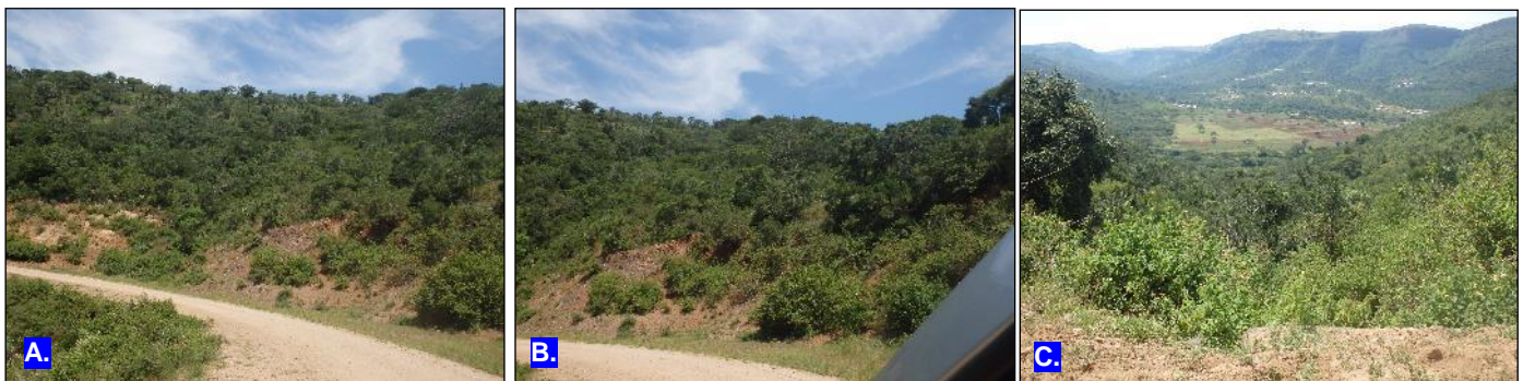
(a): Overview of RC2 adjacent to the P381 (b): Upstream of RC2. (c): Downstream of RC2.
