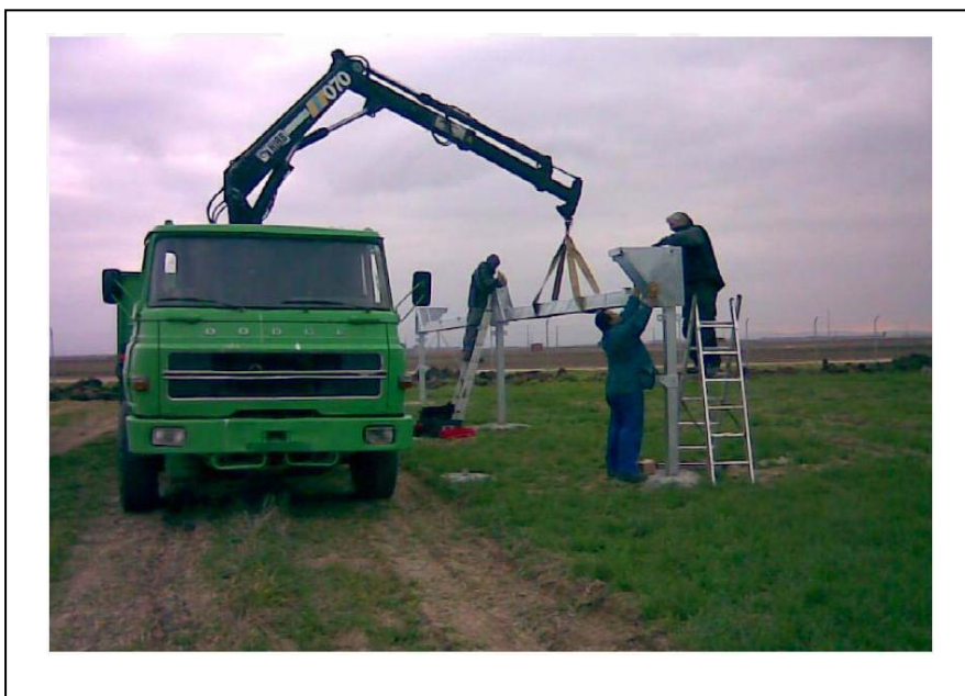
Figure 2.5 Mounting of the frame for the PV panels (Courtesy of Igeam, 2011)
