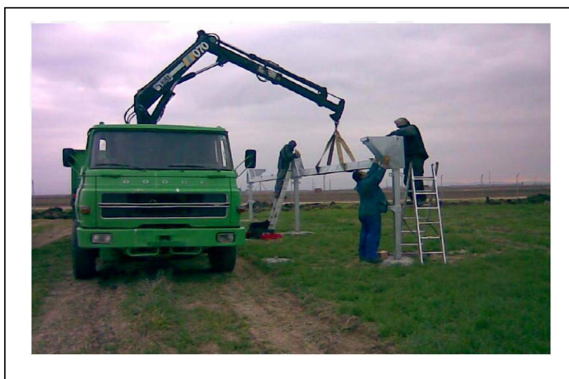
Figure 2.5 Mounting of the frame for the PV panels (Courtesy of Igeam, 2011)
