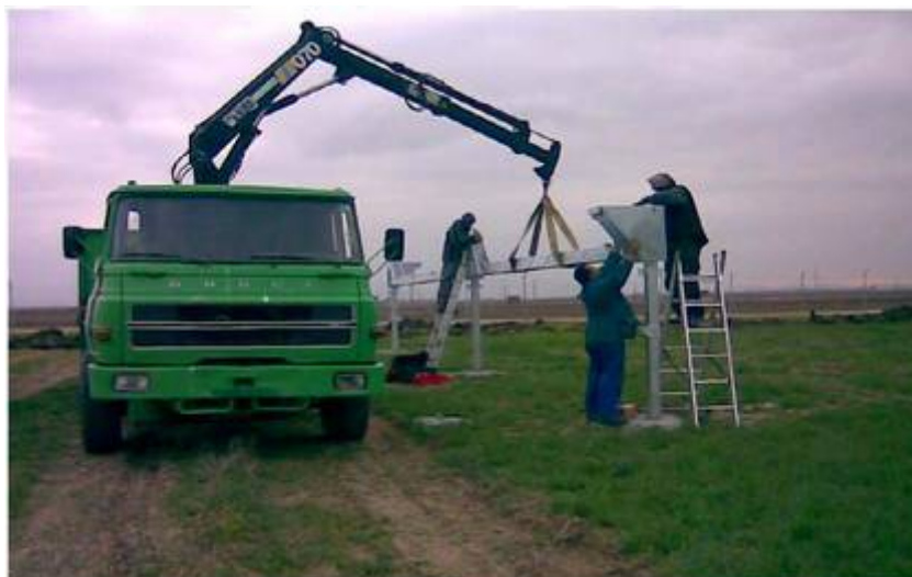
Figure 2.4 Mounting of the frame for the PV panels (Courtesy of Igeam, 2011) Inverters will be installed to facilitate the connection between the solar energy facility and the Eskom electricity grid via the proposed 132kV power line. The position of the inverters within the footprint of the broader site will be informed by the final positioning of the PV components.
