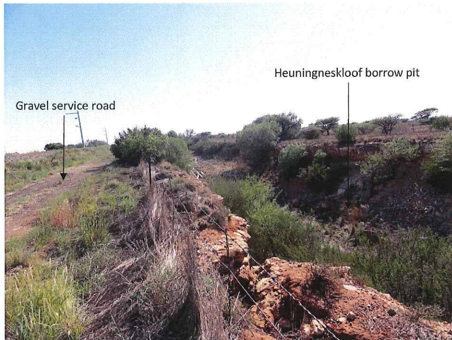
Figure A: Heuningneskloof borrow pit adjacent to the gravel service road
