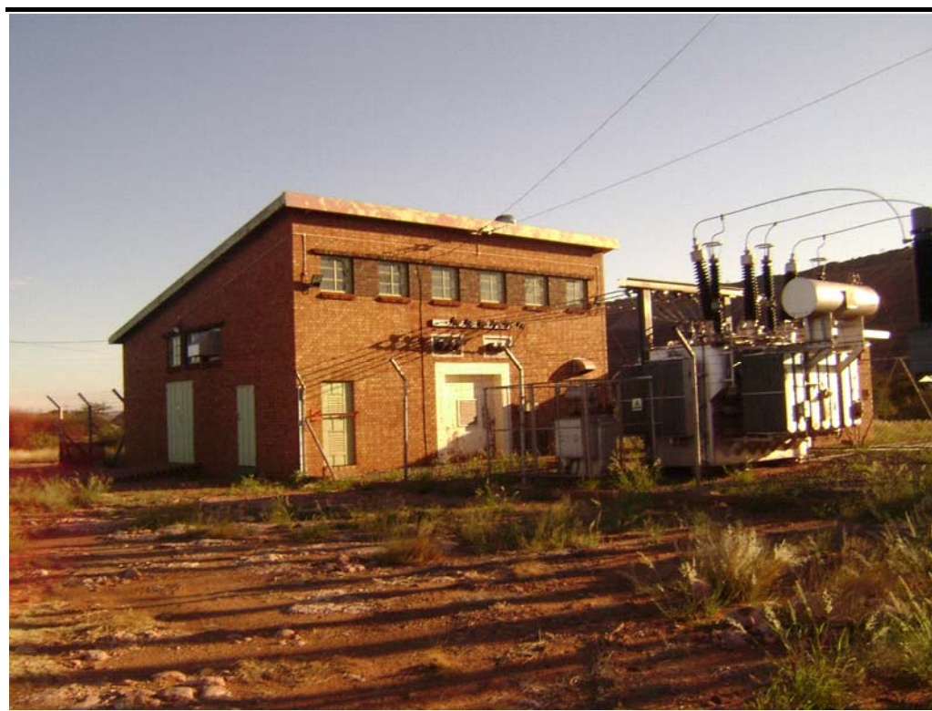
Figure 4.6 The railway related indoor equipment building (Sishen Substation)
